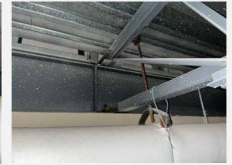
Without WinSert Interior surface temperature 116.7°
