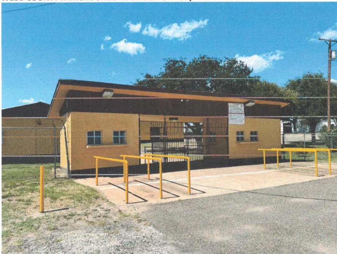
WEBB COUNTY FAIRGROUNDS MAIN BOX OFFICE / TICKET BOOTH
