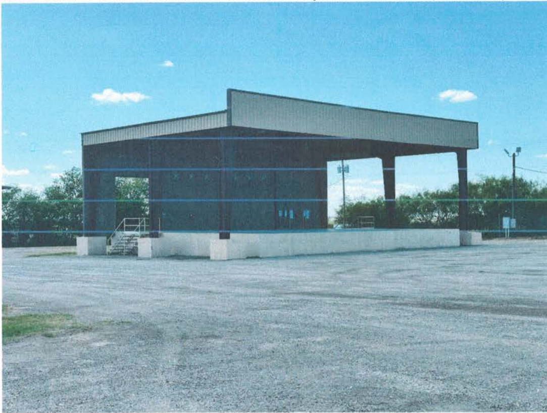
WEBB COUNTY FAIRGROUNDS STAGE STRUCTURE (APPROXIMATELY 3,850 SQ.FT.)
