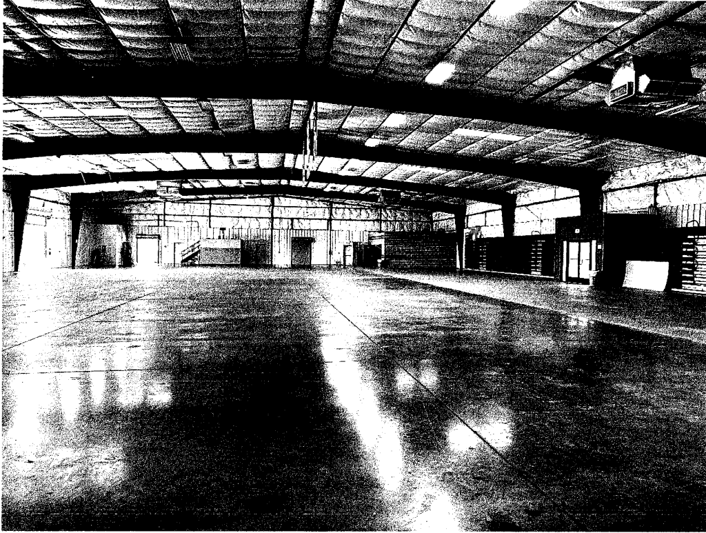
WEBB COUNTY FAIRGROUNDS INDOOR PAVILION – HVAC SYSTEM INCLUDED.
