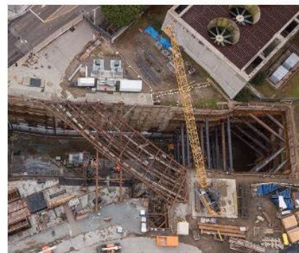
A soldier pile wall used for Regional Connector station at 2nd/Hope.
