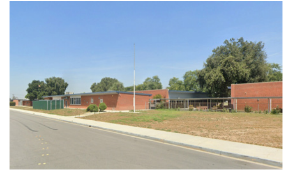
Existing W Del Norte Street and school site buildings; Specific plan area is to the right.
