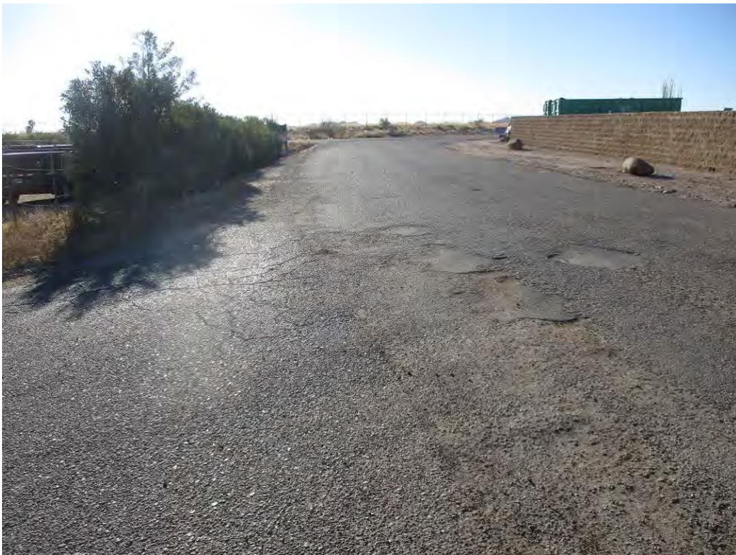
Southeast Along Industrial Drive, Subject Site At Left
