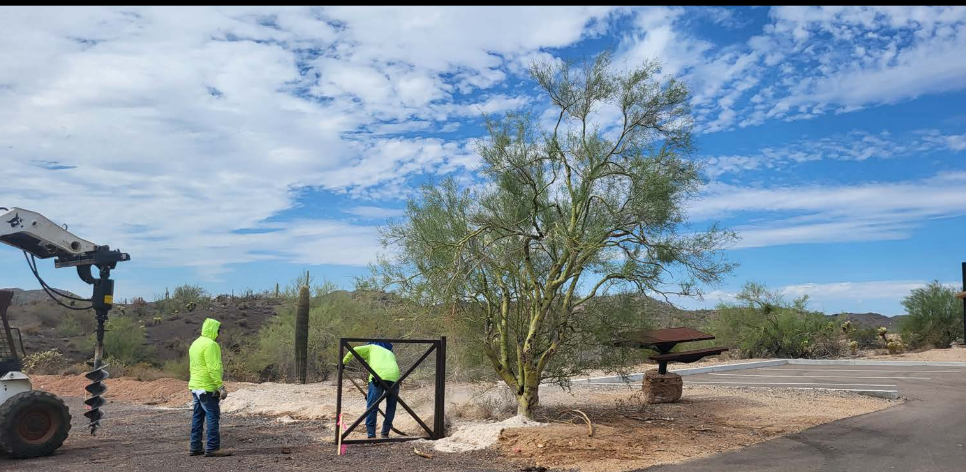
INSTALLING DECORATIVE FENCE AT DAY-USE AREA
