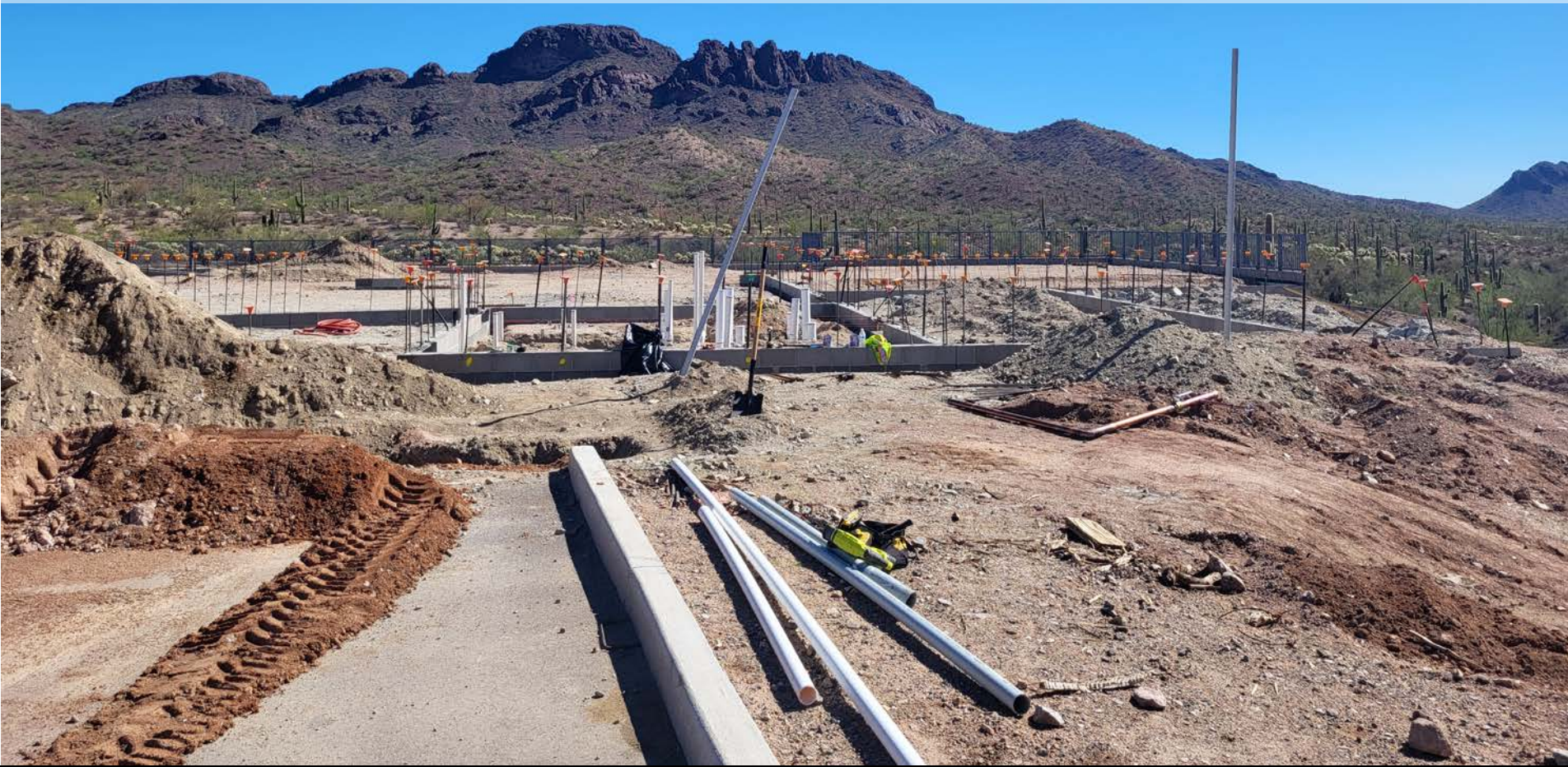
NATURE CENTER PLUMBING ROUGH IN
