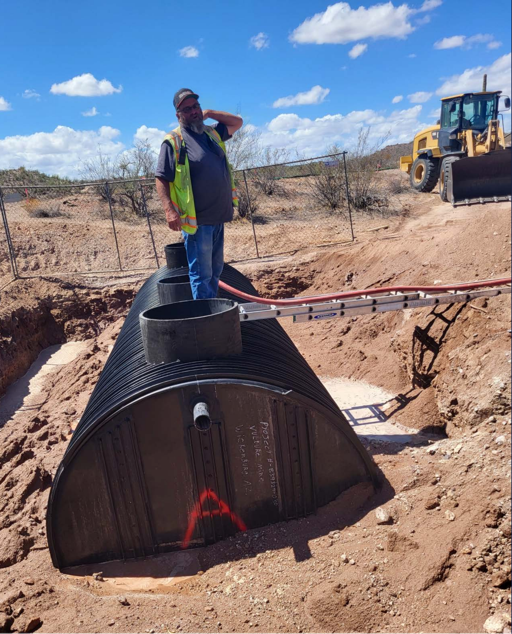
INSPECTING THE SEPTIC TANK
