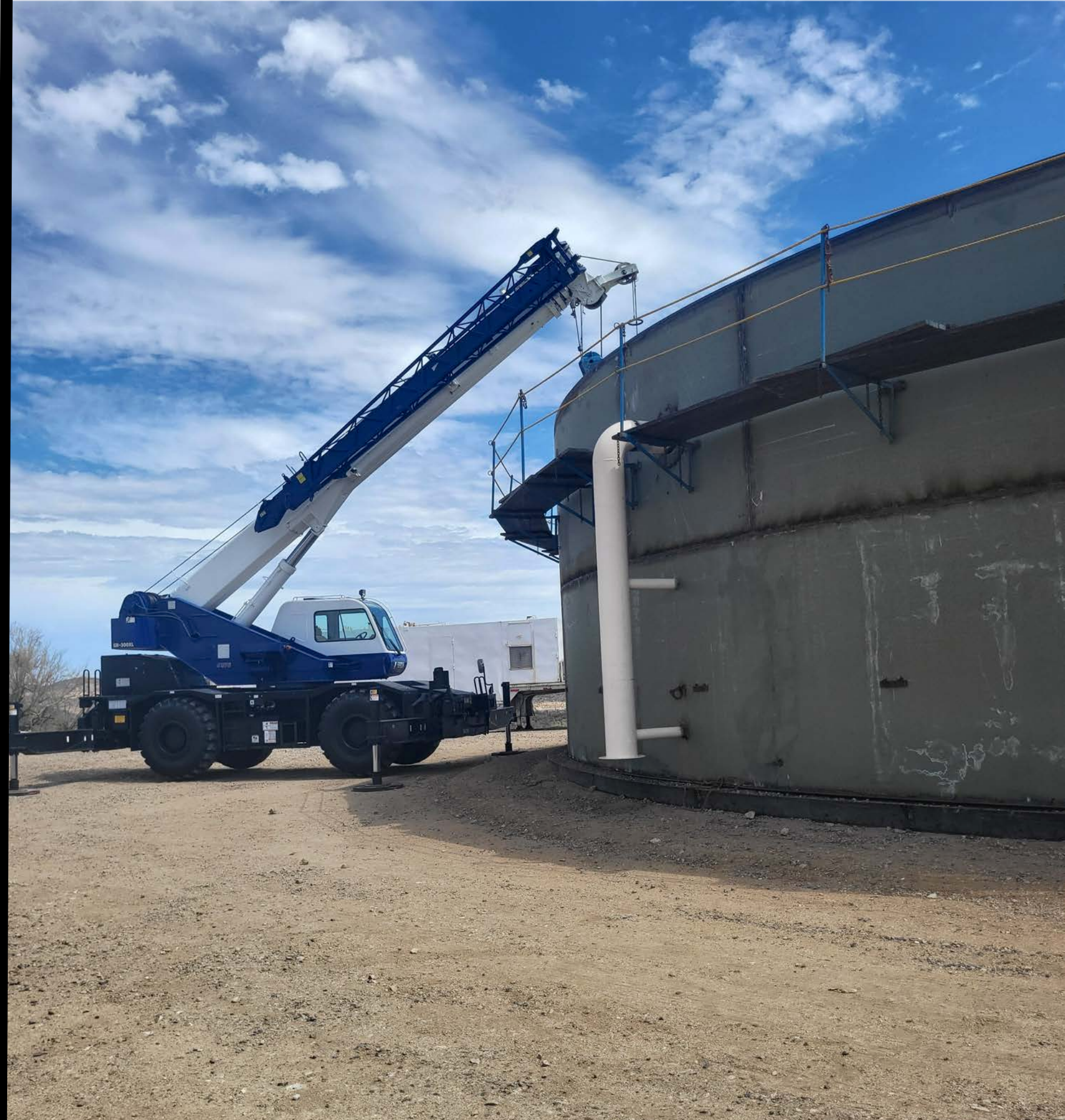
WELL SITE CONSTRUCTION
