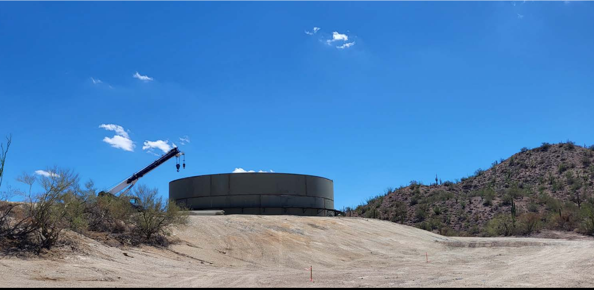
WELL SITE CONSTRUCTION
