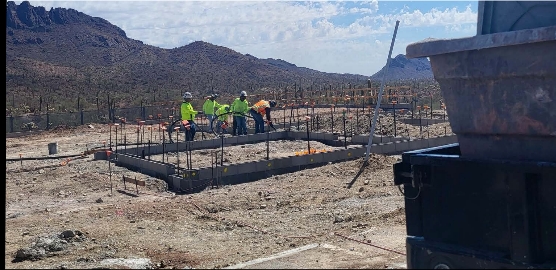
BUILDING STEM WALL FOOTINGS FOR NATURE CENTER
