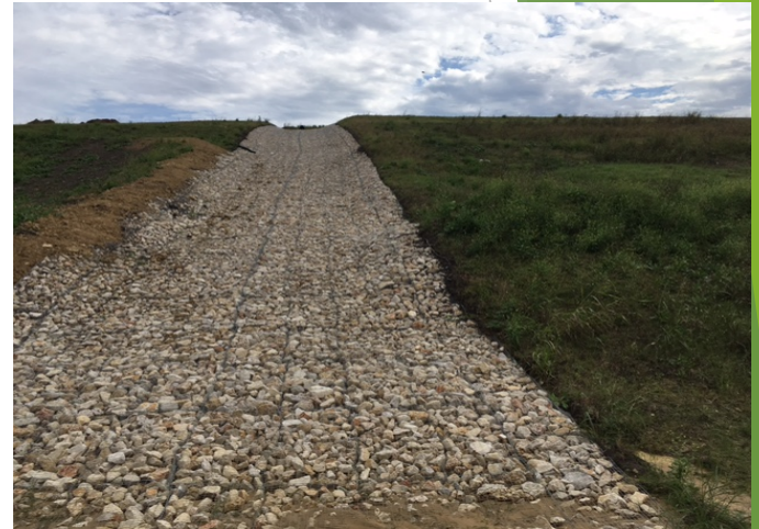
West Slope Erosion Control Drain
