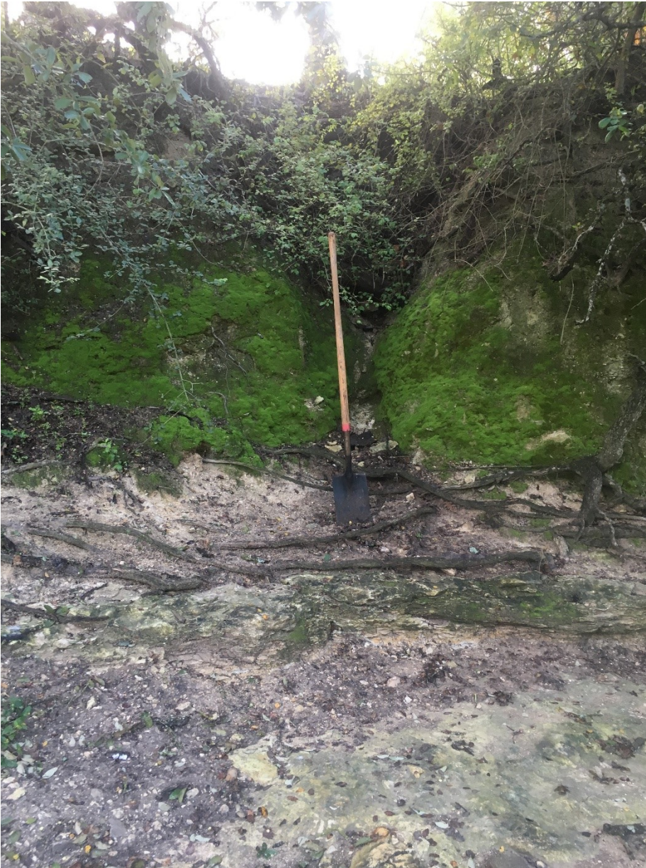
Figure 3. Profile view of Mankins Creek bank, facing south-southeast.
