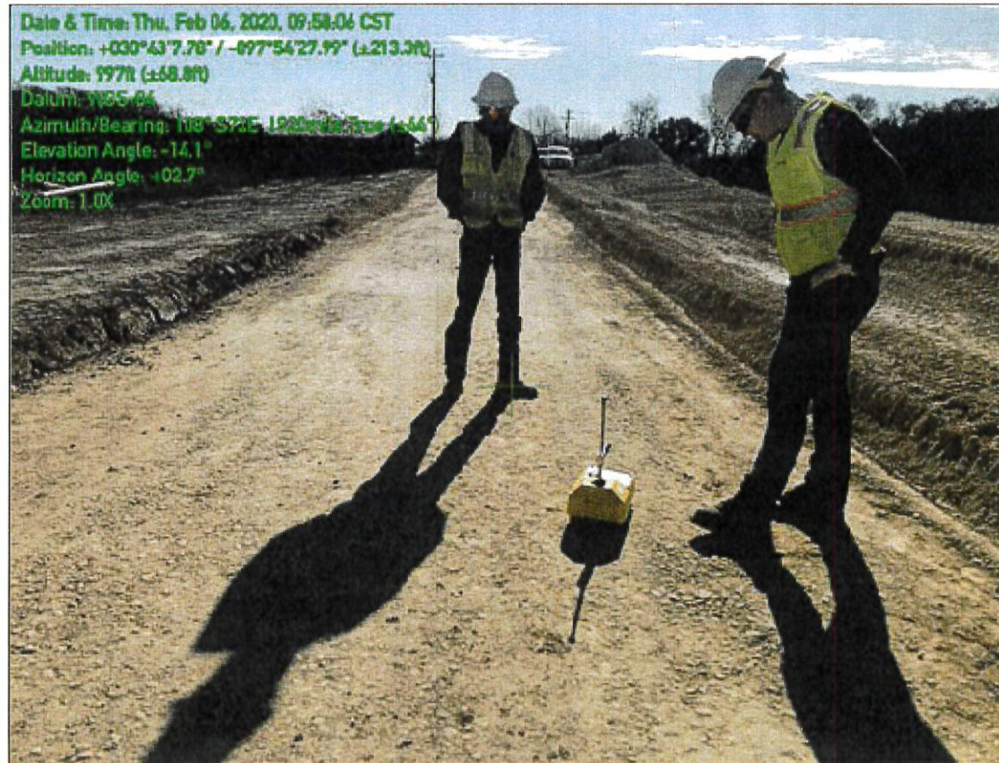
Base densities on first lift with Inspector and Kleinfelder. Densities passed.
