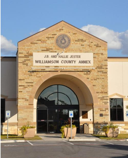
The project consisted of many different interior finishes including a formal Court Room, professional office space, kitchens/break rooms and dormitory style accommodations for the EMS staff. Exterior finishes consisted of EIFS and stone veneer with metal roofing. The buildings provide modern workspace for all employees utilizing the facilities.
