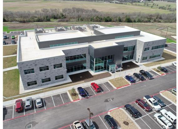
The building site is situated on a sloping site of very fat clay, so the slab was constructed as a structural pan slab with drilled piers with a perimeter grade beam to provide a voided crawl space.
