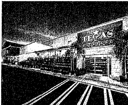
Military and Goliad H-E-B Addition and Renovation
