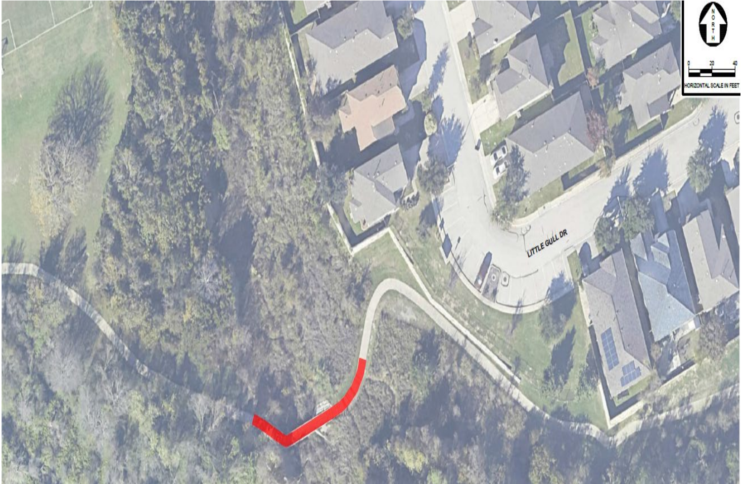
Lake Creek Trail Rip-Rap Abutment Repair
