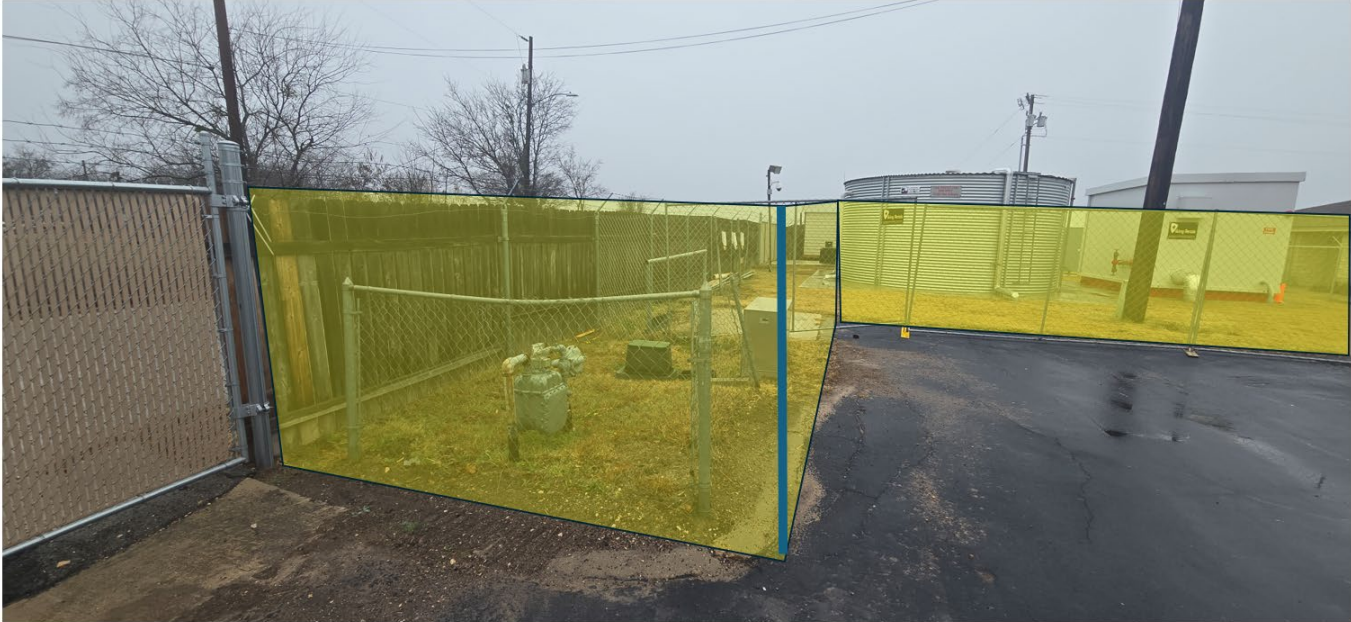
Fence Perimeter View 3 (Corner tie-in around PRV and Gas Meter)
