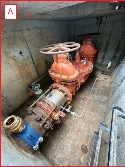
4" TAPPING SADDLE 4" BYPASS 12" GATE VALVE 12" PRESSURE REDUCING VALVE 12" GATE VALVE
