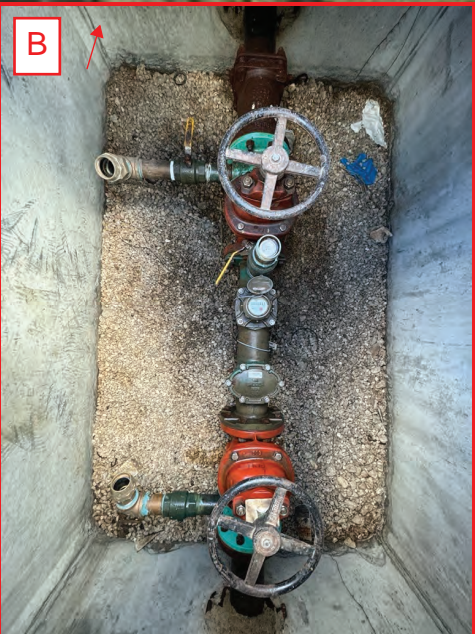
4" TAPPING SADDLE 4" GATE VALVE 4" GATE VALVE 4" METER 4" GATE VALVE 4" TAPPING SADDLE
