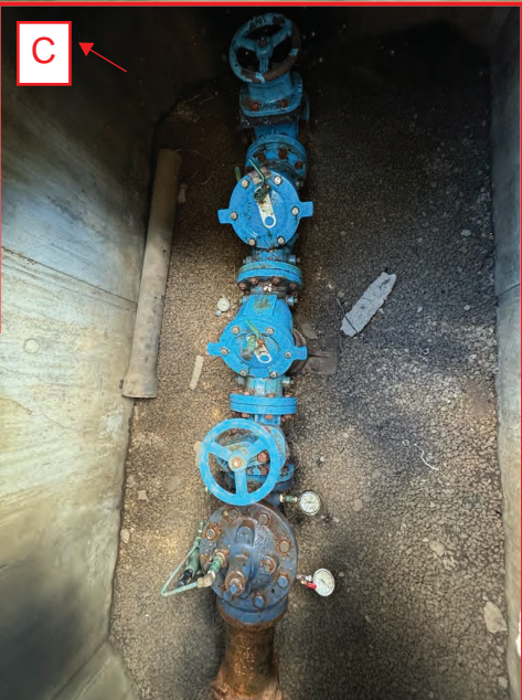
4" GATE VALVE 4" BACKFLOW PREVENTER 4" GATE VALVE 4" PRESSURE REDUCING VALVE
