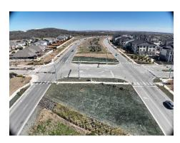
Description of Project: 1.2 miles of E. William Cannon Dr. This project included the west bound side of the roadway with its terminus at the existing intersection of US 183 & FM 1625. The project included the base and paving, multi-barrel box culverts, MSE walls, waterline install, type 'C' embankment, curb, sidewalk and all other roadway construction.
