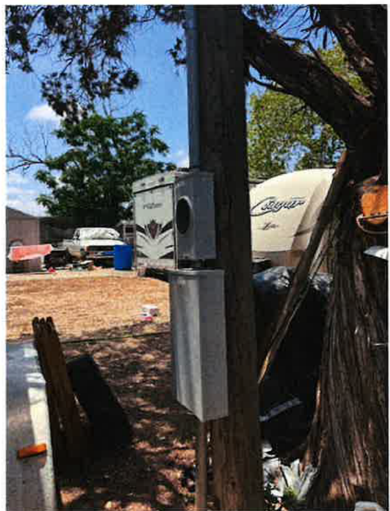
New meter box attached to pole on remainder
