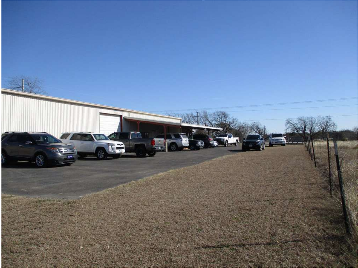
Southern Elevation of of Office/Warehouse Building:
