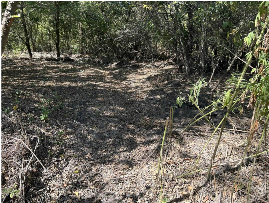
Photograph 4 (PP04): View of erosional feature into W-1A, facing northwest.
