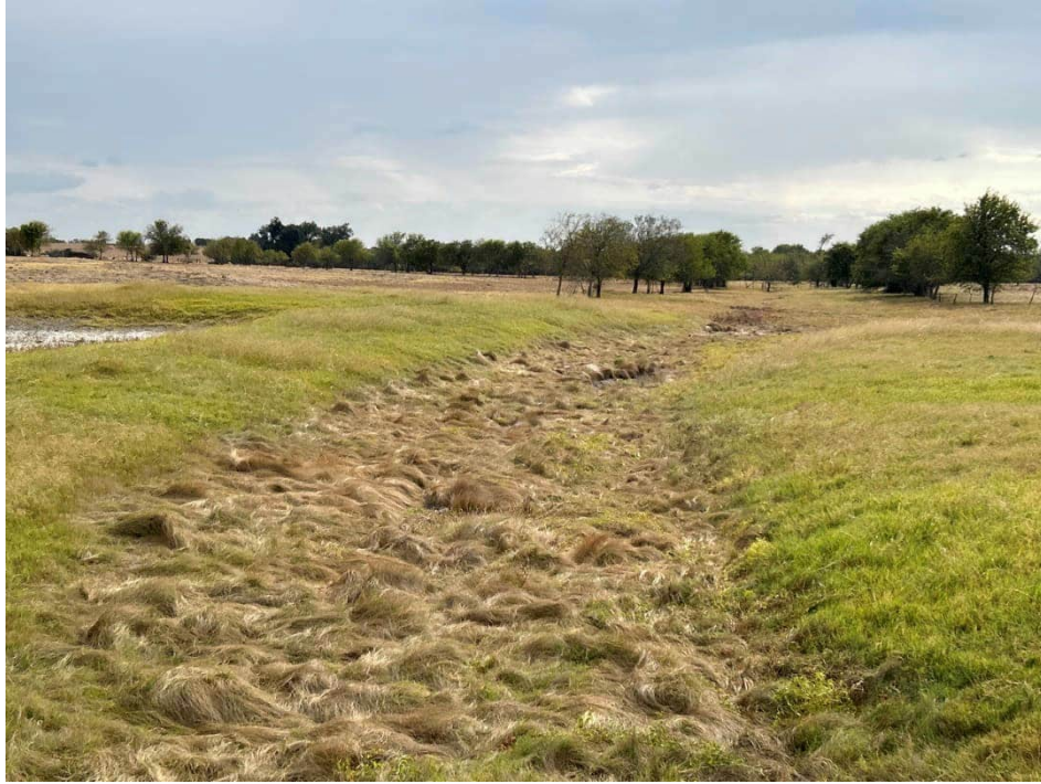
Photograph 13 (PP13): View of vegetated swale (W-4), facing downstream and southwest.
