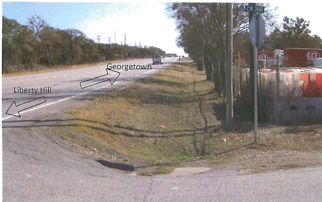
Figure 16. Existing Condition: CR 266
