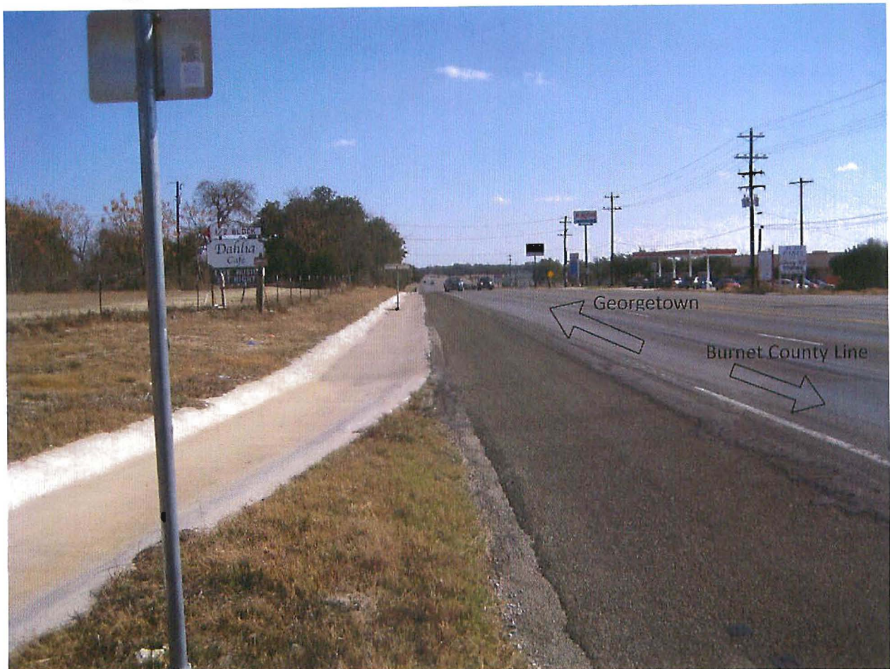
Figure 13. Existing Conditions: FM 1869
