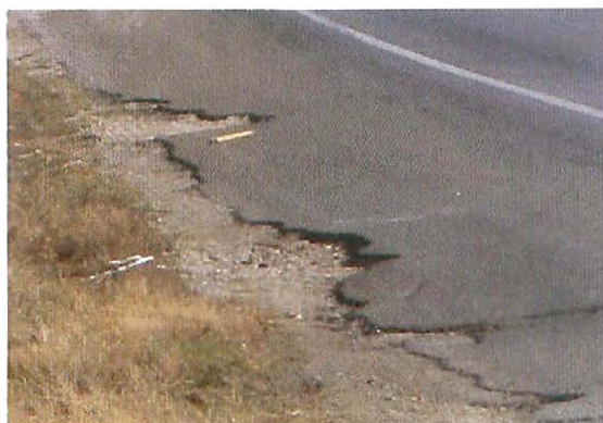
Figure 7. Existing Condition: Liberty Hill City Limit Shoulders
