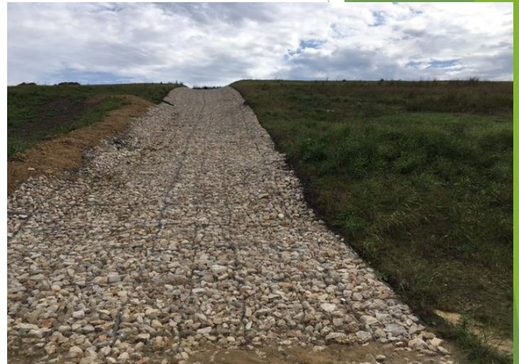
West Slope Erosion Control Drain
