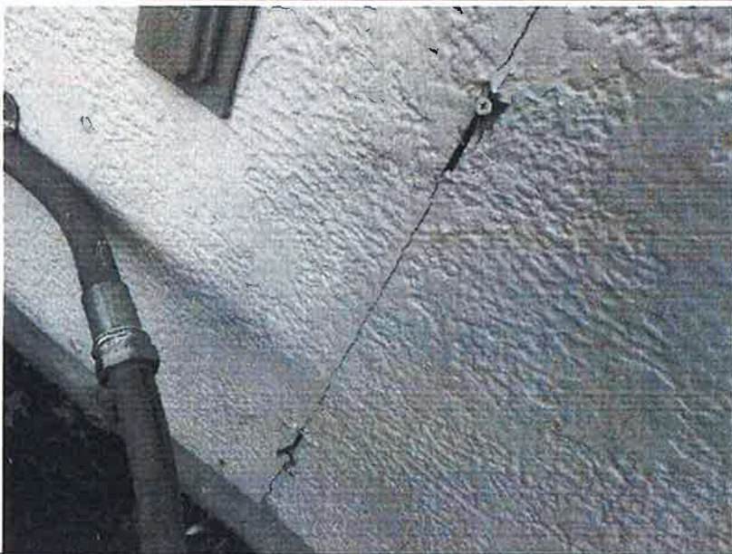
Photo No. 2 Example of damaged siding.
