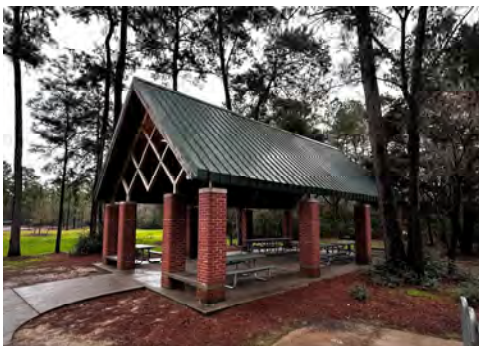
Falconwing Pavilion Renovation Before and After
