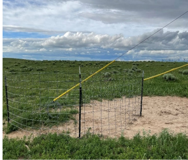
Figure 7. Cattle Fencing Around Guy-Wire Anchor
