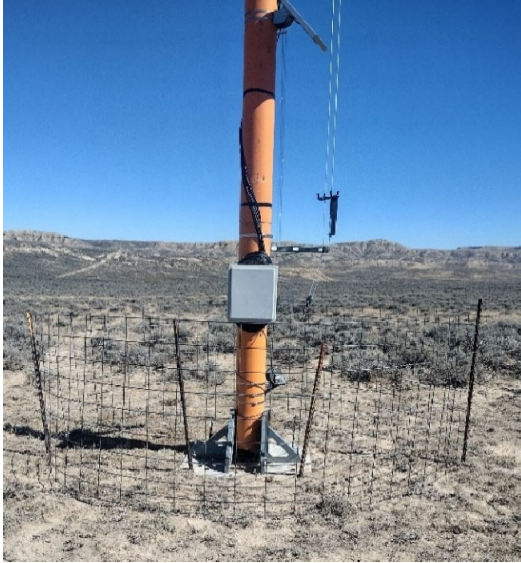
Figure 6. Cattle Fencing around Met Tower Base
