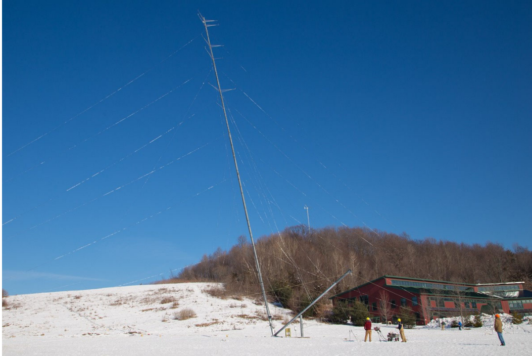
Figure 4. NRG Systems 60-meter XHD Tall Tower – Example of Installation Process
