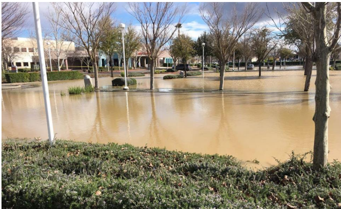
Sutter-Davis Hospital during the 2019 flood, showing no access to the parking lot.
