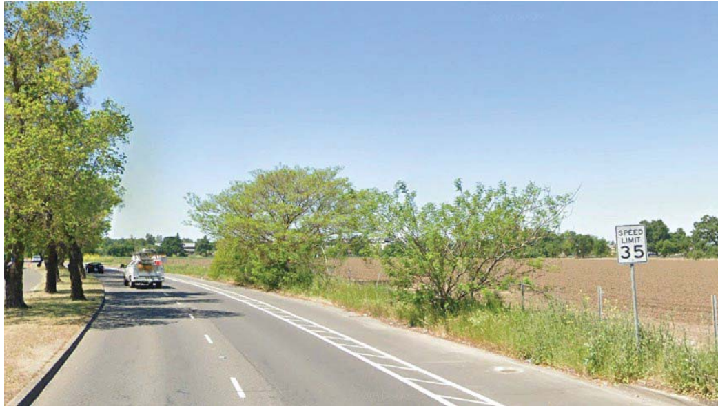
Figure 6-Example of a buffered Class II bike lane on Covell Blvd in Davis, Ca
