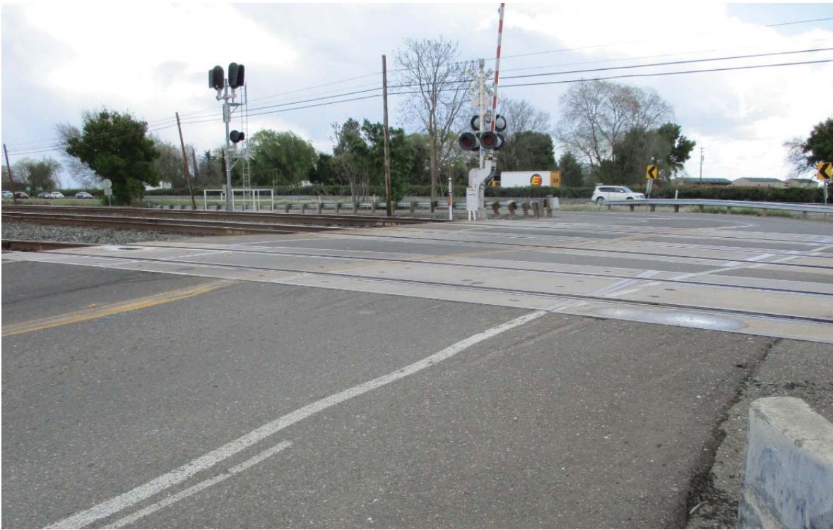
Photo of the at-grade UPRR crossing at CR 32A and CR 105
