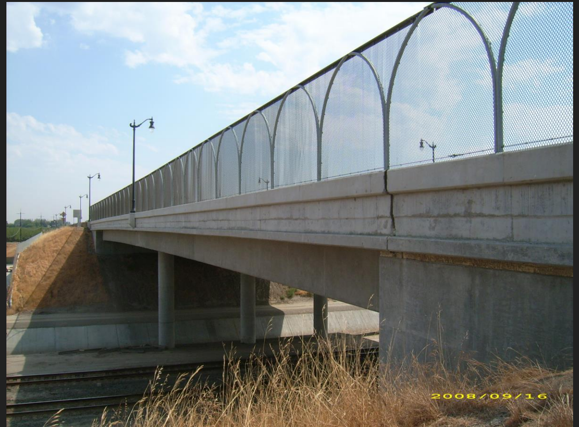
Similar Grade Separation Project in Lathrop, CA
