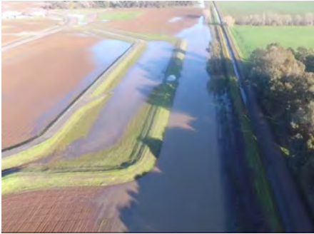
Airport Drainage Basin
