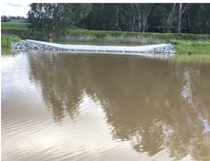
Airport Drainage Basin
