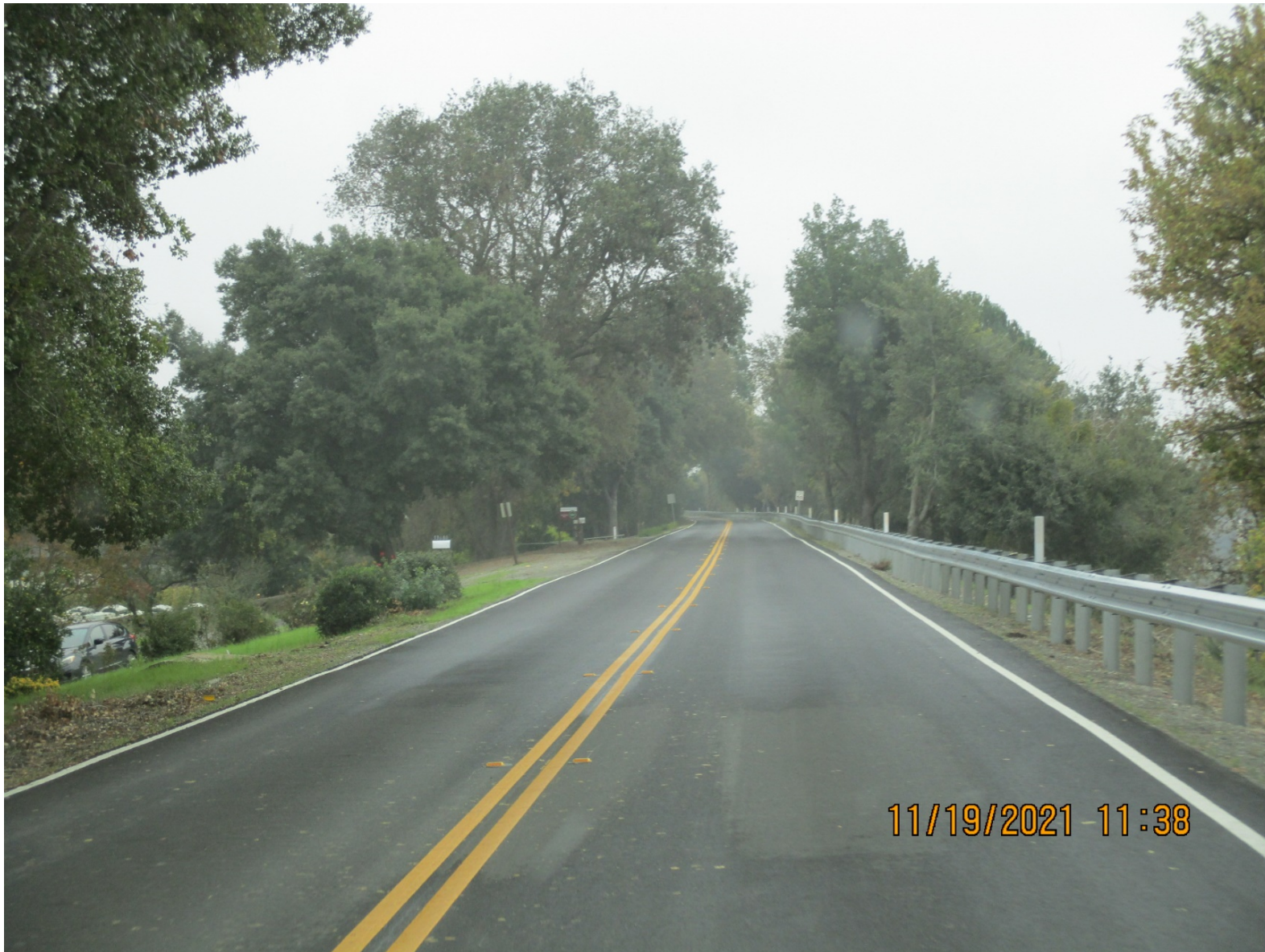
South of Freeport Bridge South River Road, Guardrail and Cape Seal – Photo 2
