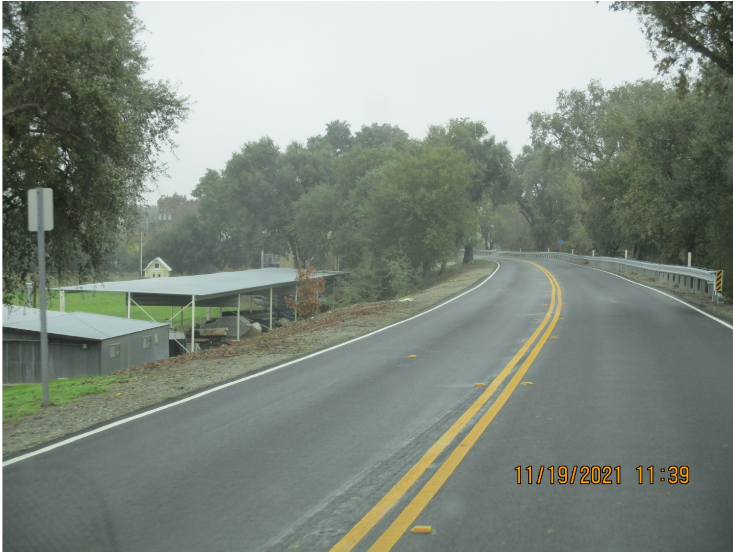
North of Freeport Bridge South River Road, Guardrail Cold in Place Recycle with new Asphalt – Photo 3
