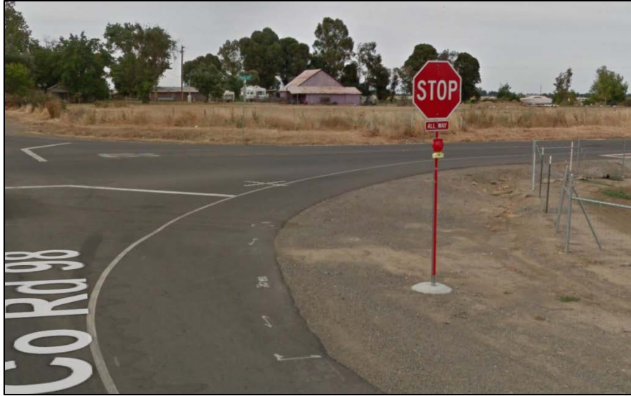
Figure 1 - All red reflective striping down entire length of stop sign posts for enhanced visibility / reflectivity
