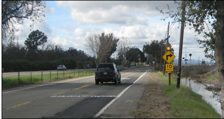
Figure 5 – Warning rumble strips and flashing beacon ahead of Co Rd 32A & Co Rd 105 with Union Pacific/Amtrak at-grade crossing.
