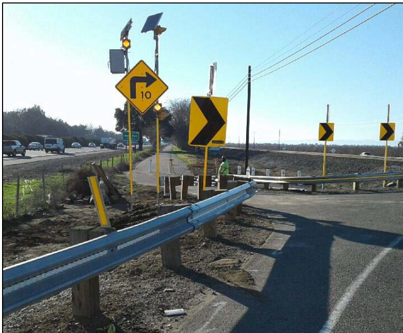
Figure 4 - Warning beacon lights and chevrons at Co Rd 32A curve before Union Pacific/Amtrak crossing
