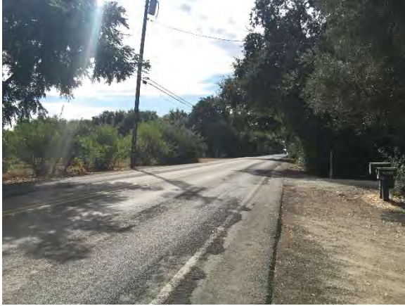
Looking southeast at County Road 98.
