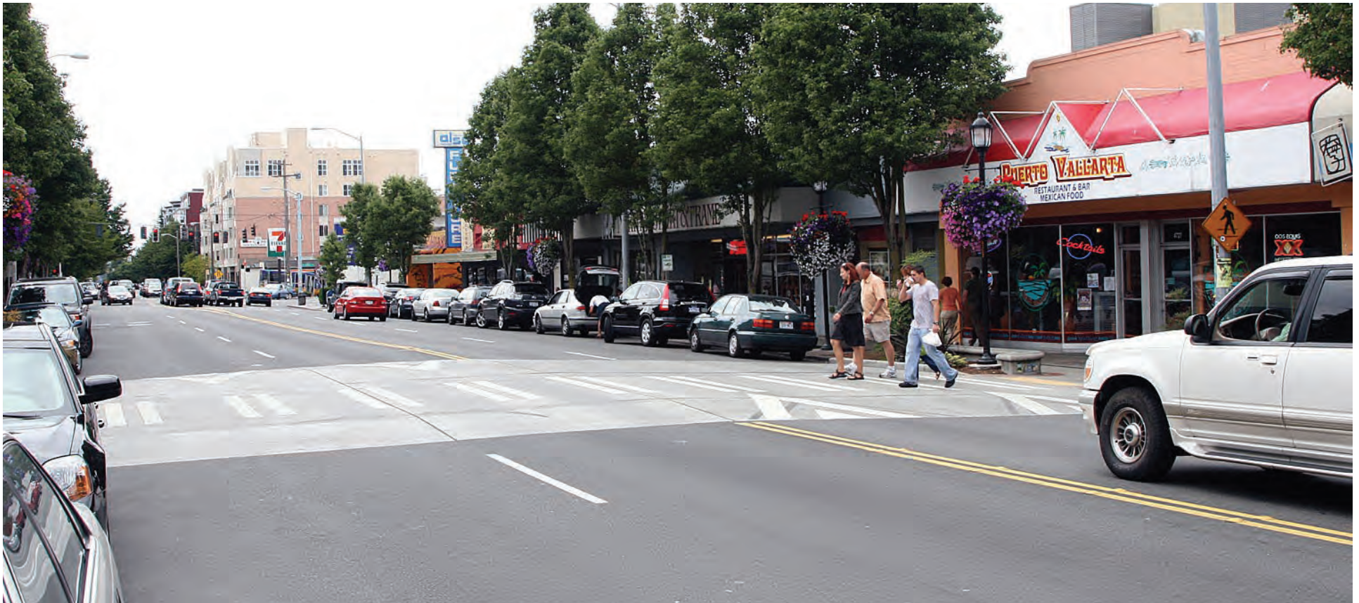
Raised Crosswalk in Seattle, WA
