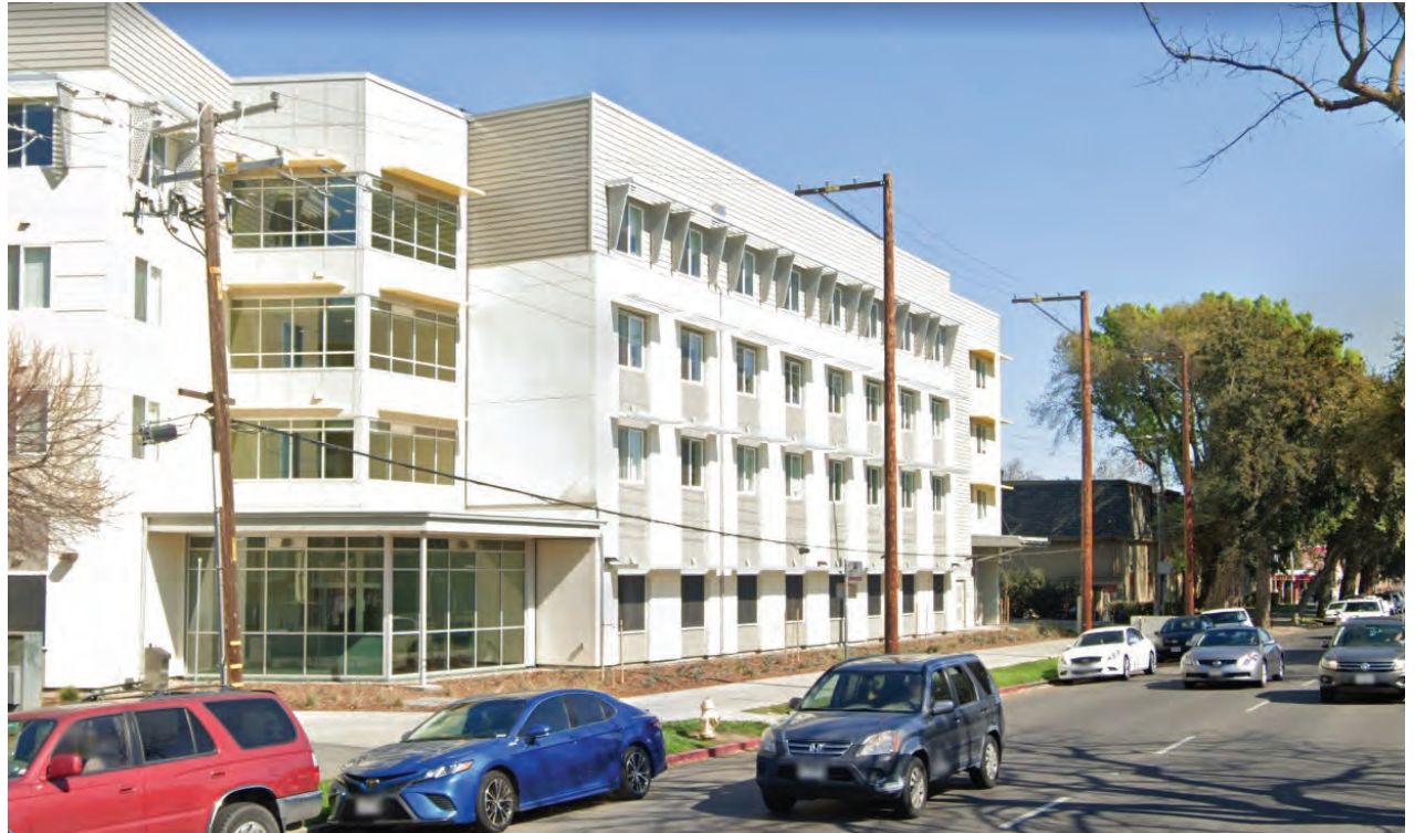
Overhead Wires at Yosemite Hall
