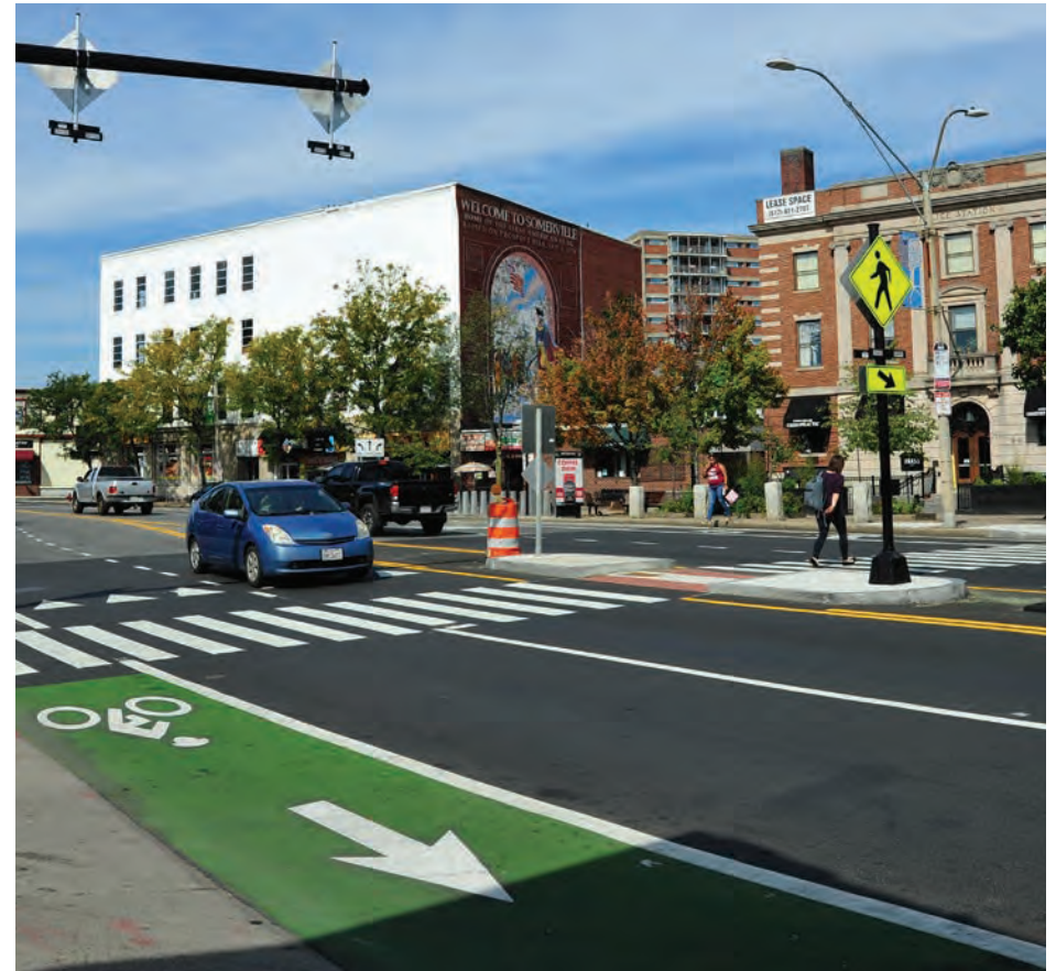
Mid-block Crossing with Pedestrian Refuge Island in Somerville, MA
