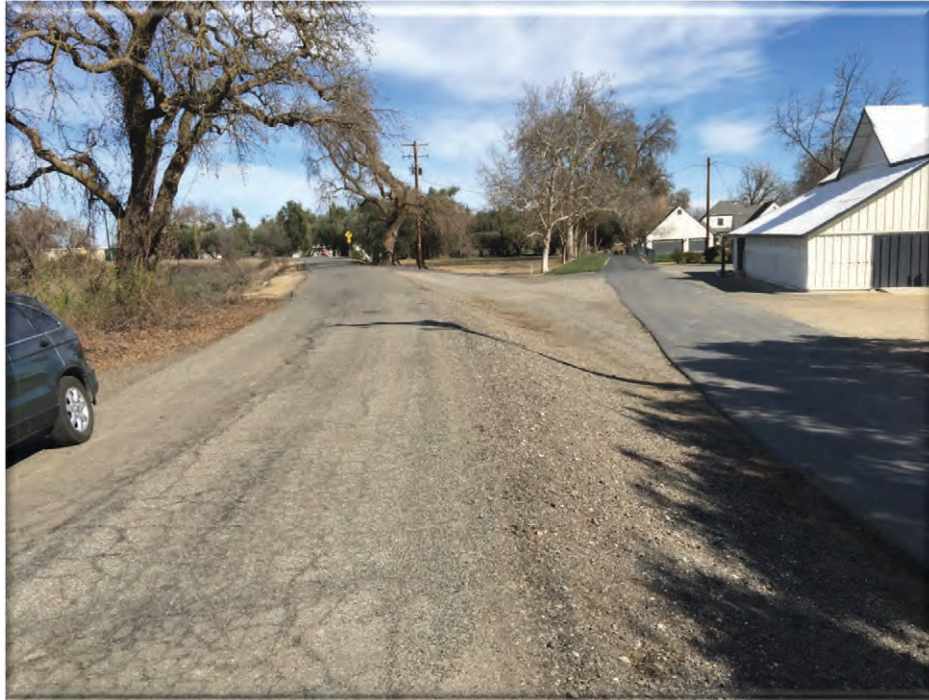
Plate 3. Looking east along County Road 18. The levee rehabilitation project extends from the north shoulder of the road (left side of photo) to approximately 40 feet south of the south shoulder.
