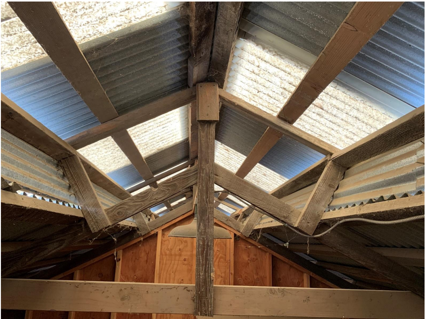
Figure 28: Interior view of the monitor roof and skylights of the Barn, showing generally original framing elements and workmanship. Photo by Lyn Hooper, 2020.
