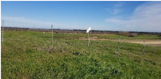
Photo 3: PG&E pipeline alignment at Location A. Taken facing east.
