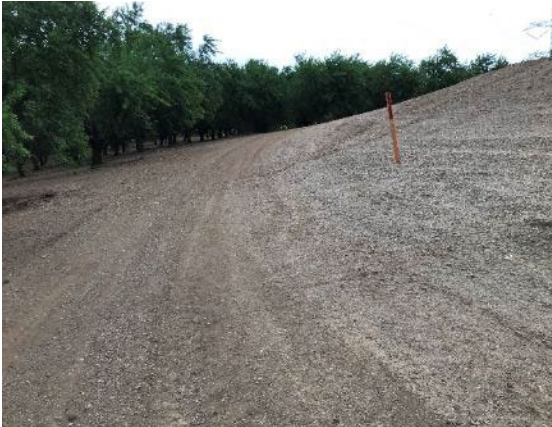
Photo 1: Wire 02.1 Start location in almond orchard. Taken facing east.
