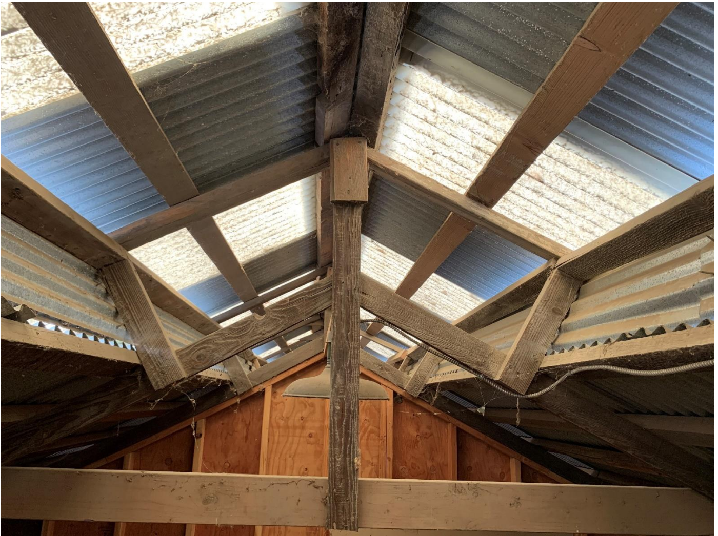
Figure 28: Interior view of the monitor roof and skylights of the Barn, showing generally original framing elements and workmanship. Photo by Lyn Hooper, 2020.
