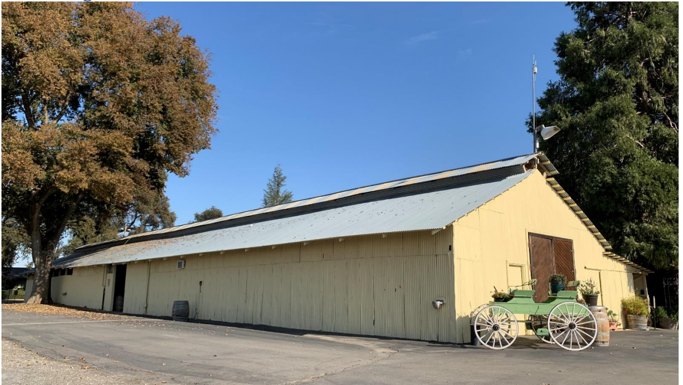
Figure 26: West and South façades of the Barn at Utter Ranch, looking northeast. Photo by Lyn Hooper, 2020.
