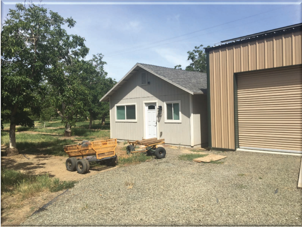
Plate 1. 820 square foot structure on the west side of the barn.
