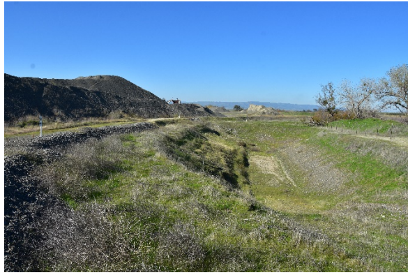
Westernmost stormwater basin, at north side of site, looking west. Cache Creek levee visible on right side of photo.
