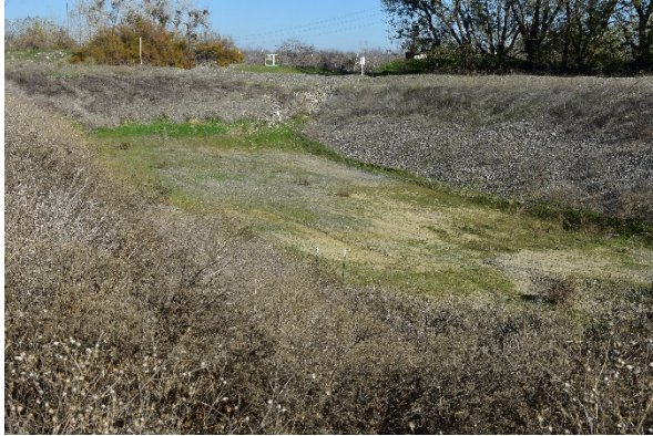
Easternmost stormwater basin, looking northeast toward CR89, showing recent cleanout/maintenance activity.
