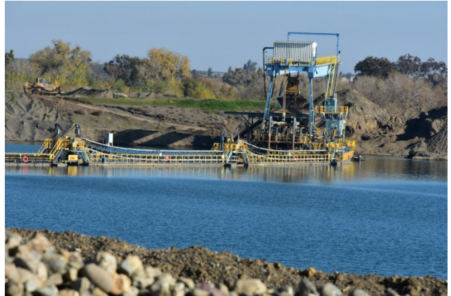
Floating Dredge – looking north from south edge of wet pit
