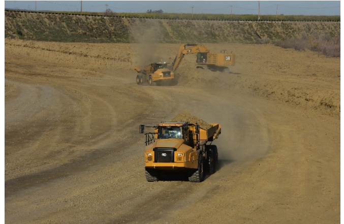
Removing overburden for future mining – looking north
