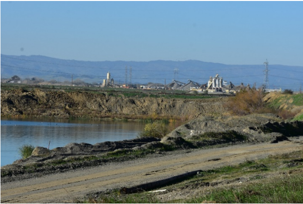
Cemex Plant site & equipment – looking west from wet pit
