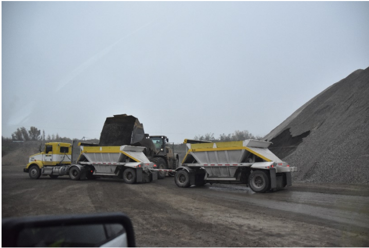
Aggregate loaded from stockpile for transport to project site
