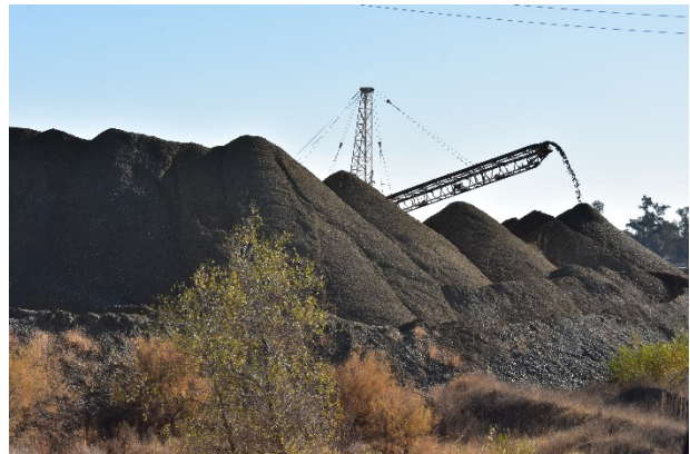
Woodland Plant Site (active) looking east, showing stockpiles of material
