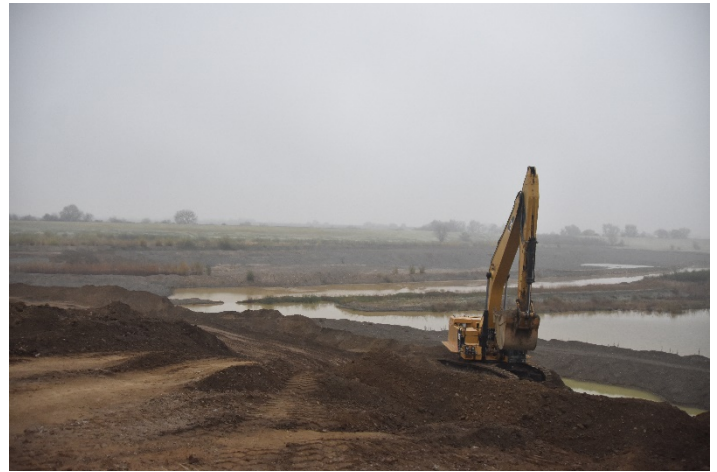
Mining with excavator – south side of Schwarzgruber pit
