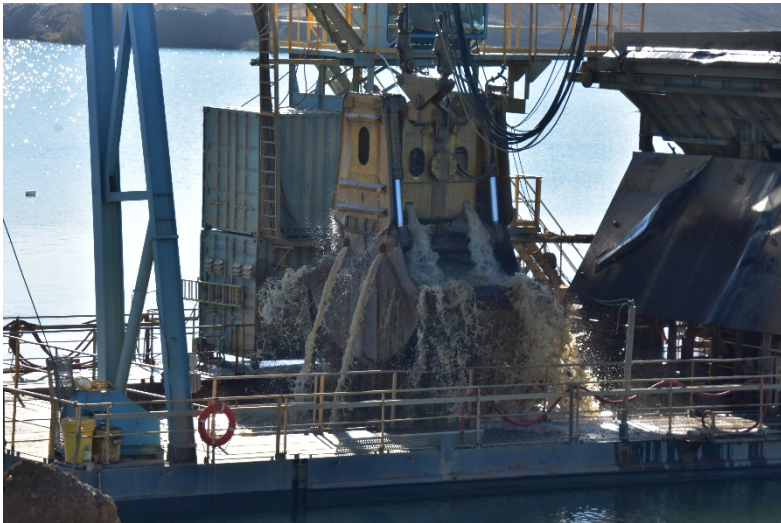
Floating Dredge – active mining - closeup
