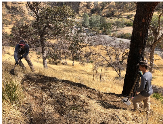
Tuleyome contractor, Kyle Lewald (right) directing construction of switchback on Oct 22
