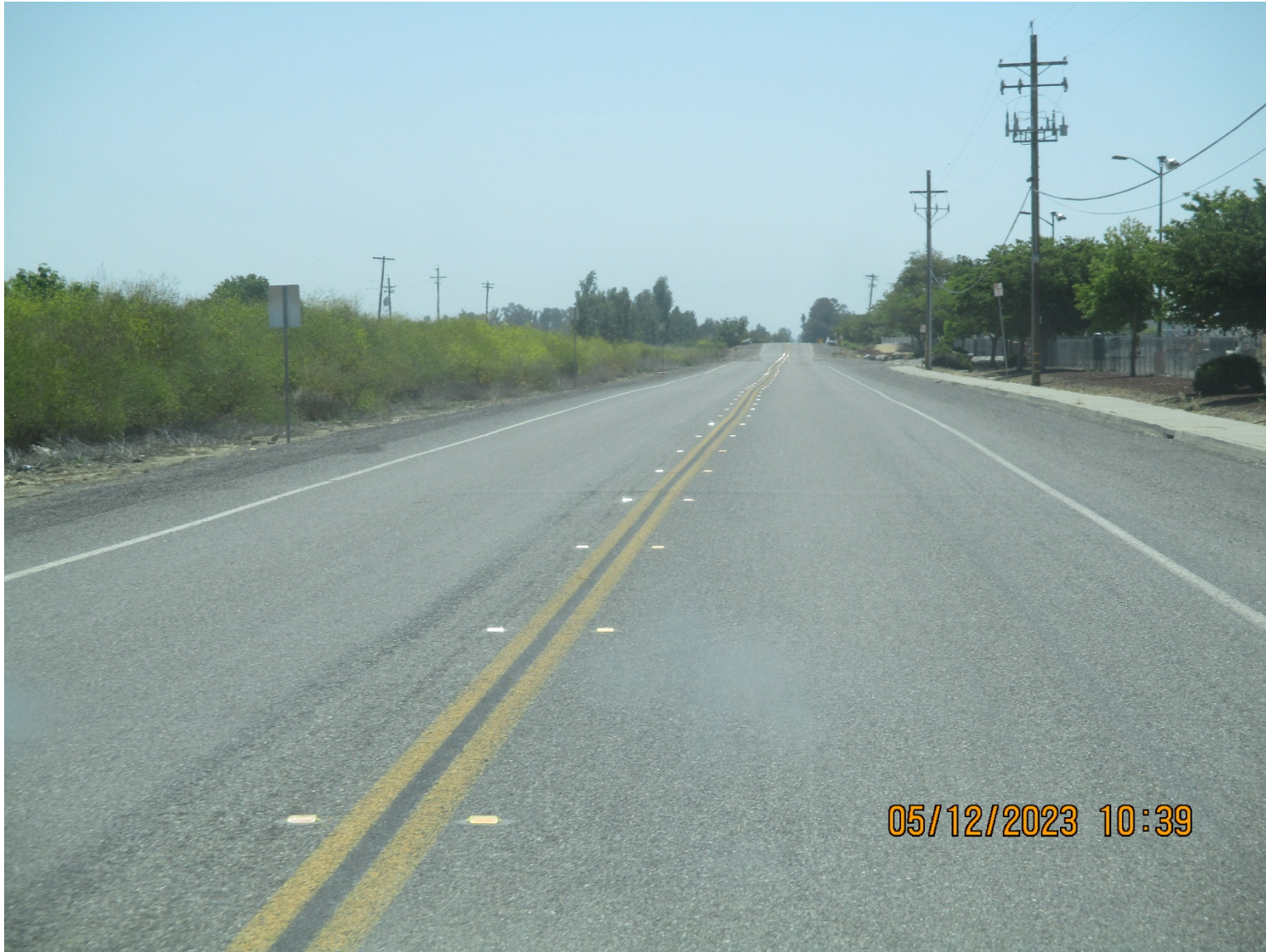
CR 99W Pavement Rehab – Photo 3
