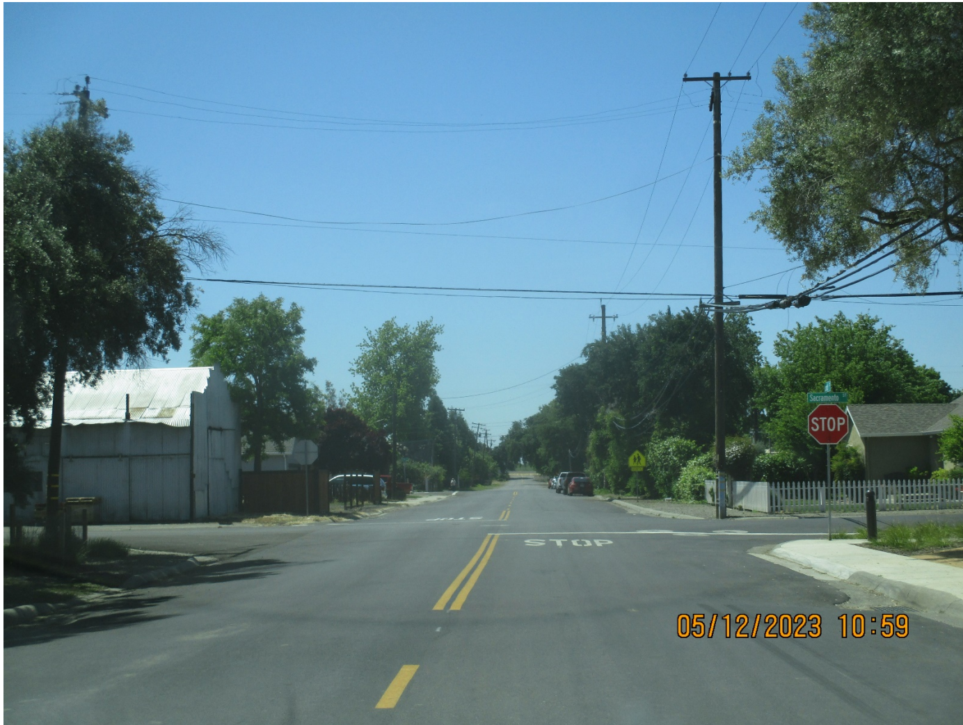
Yolo, Pavement Rehab – Photo 1
