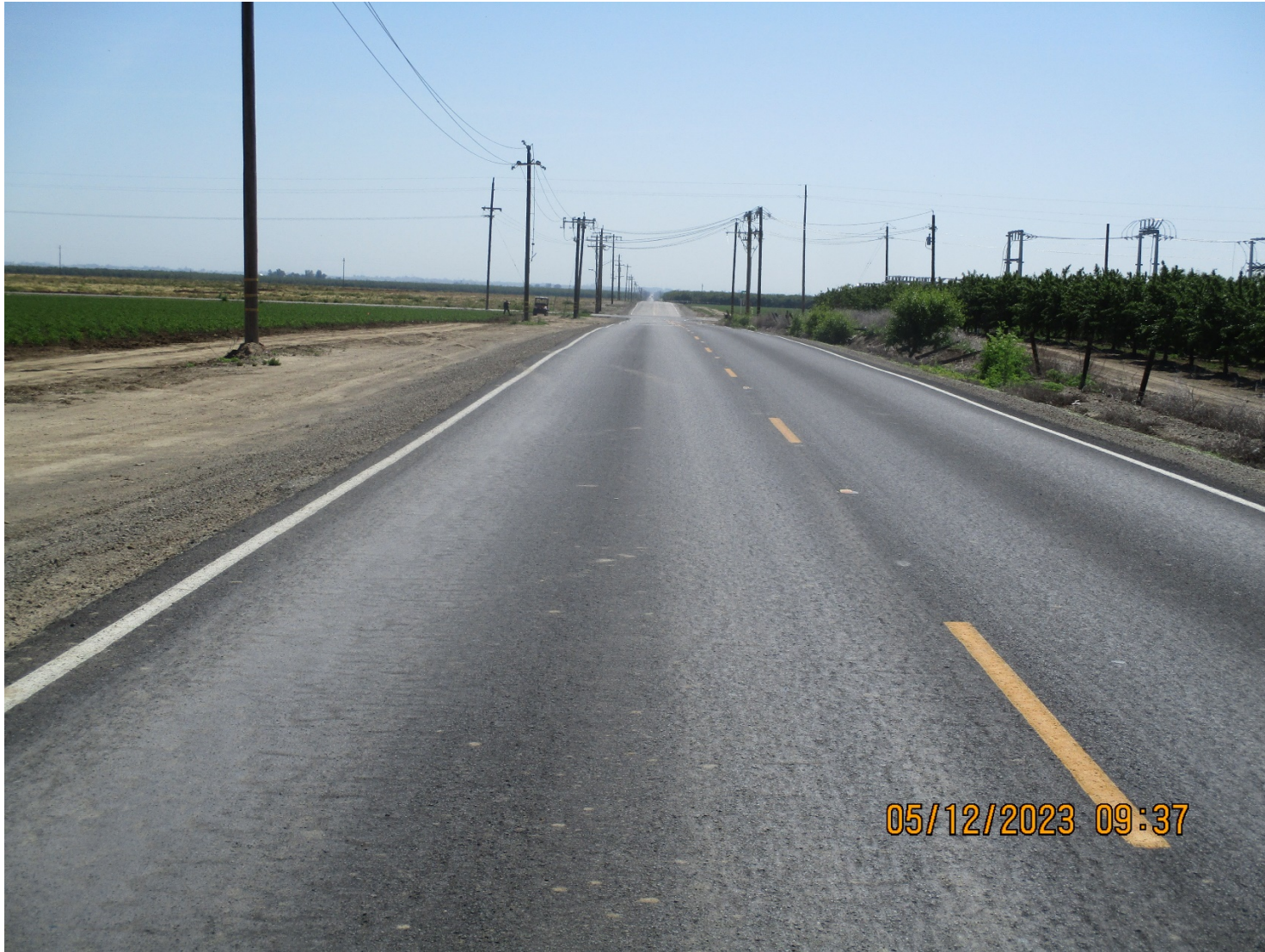
CR 99W Pavement Rehab – Photo 2
