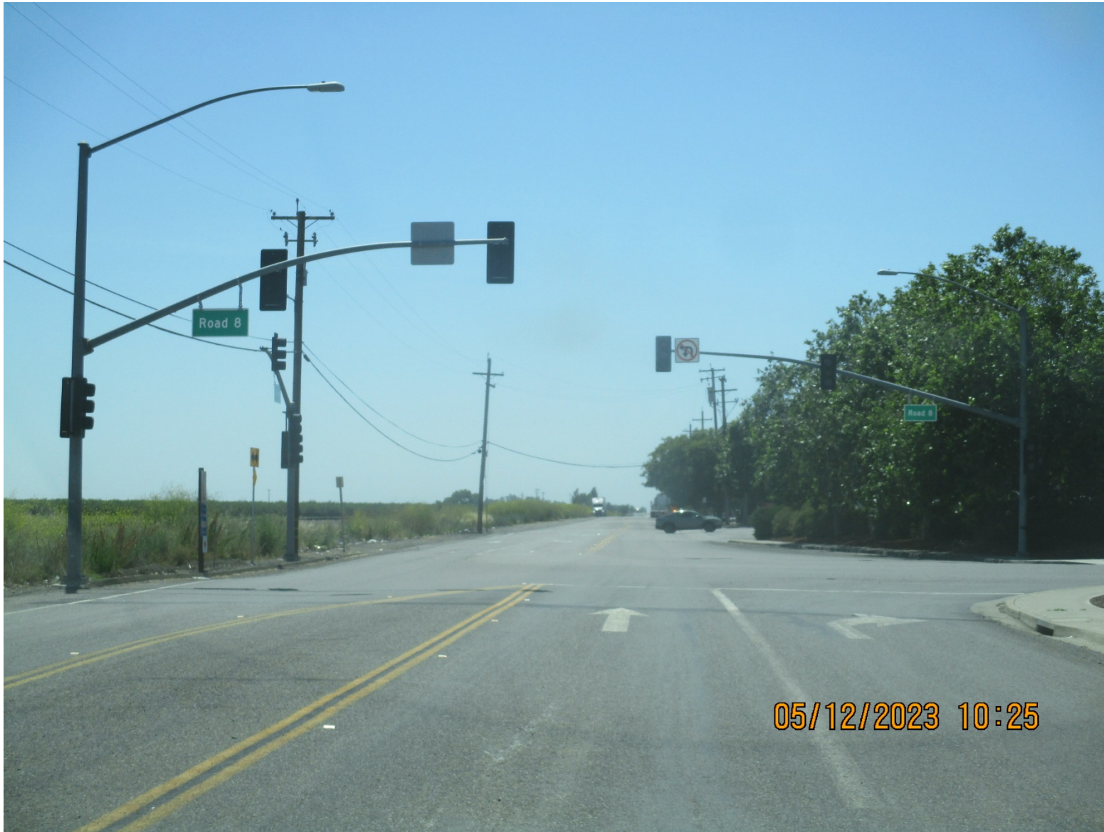
CR 99W AT CR 8 Intersection pavement repair- Photo 6
