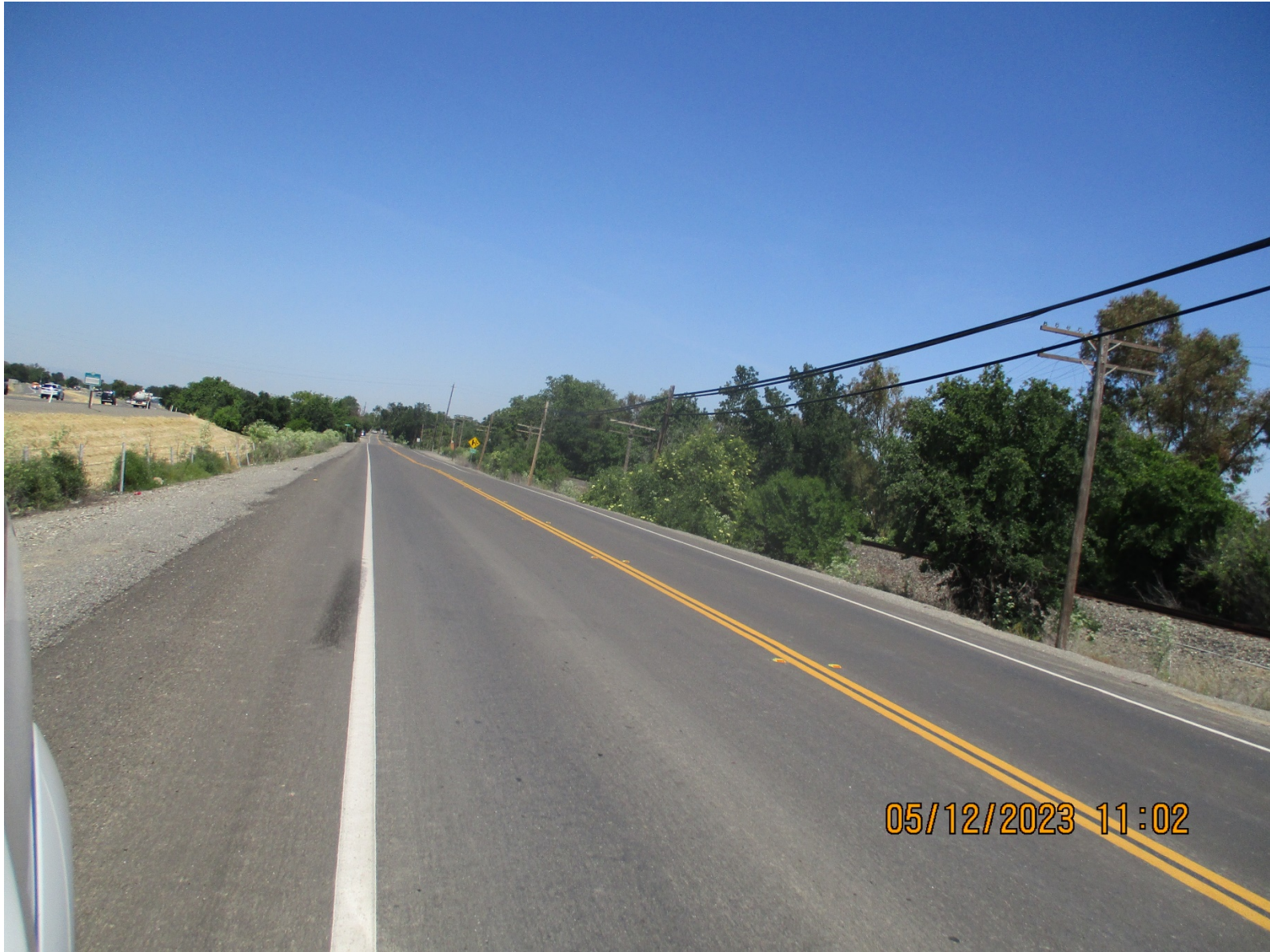
CR 99W Pavement Rehab – Photo 5
