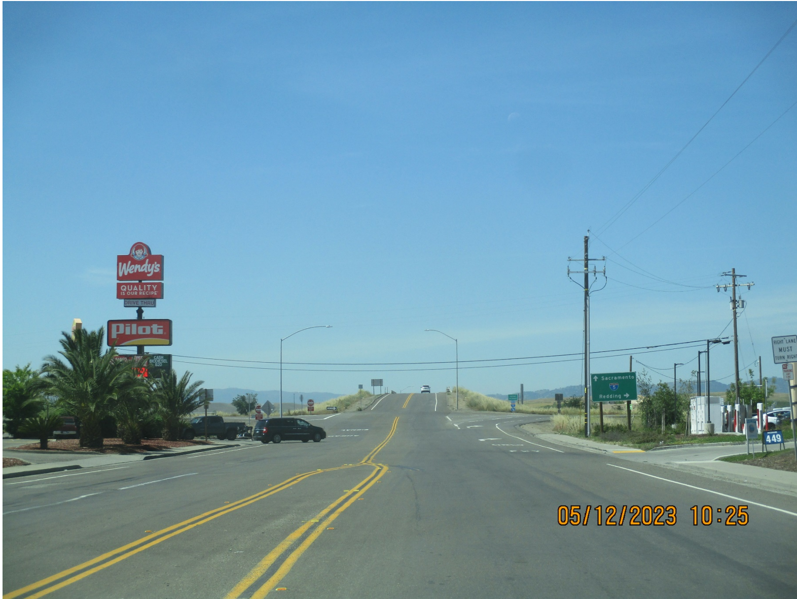
CR 8 Pavement Rehab– Photo 4
