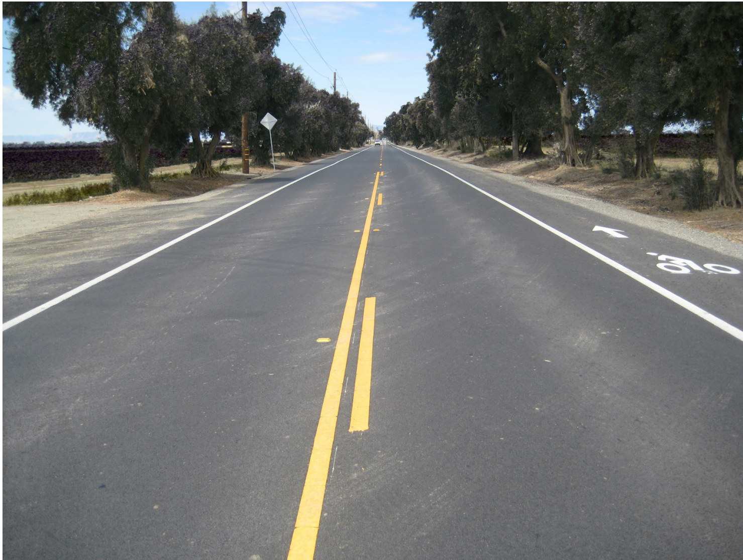
CR 27, Bike Lane & Road Rehabilitation – Photo 1
