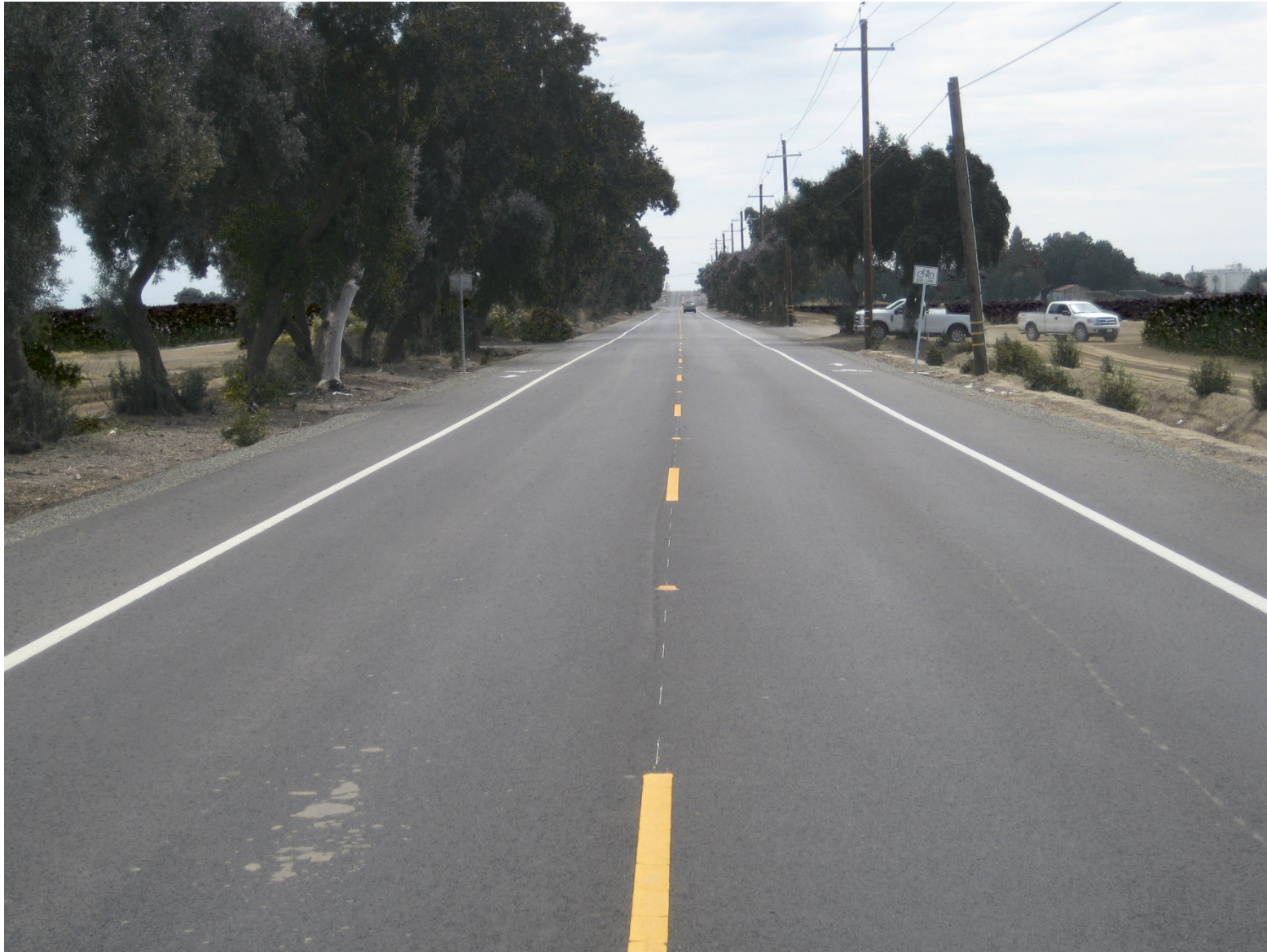
CR 27, Bike Lane & Road Rehabilitation – Photo 2
