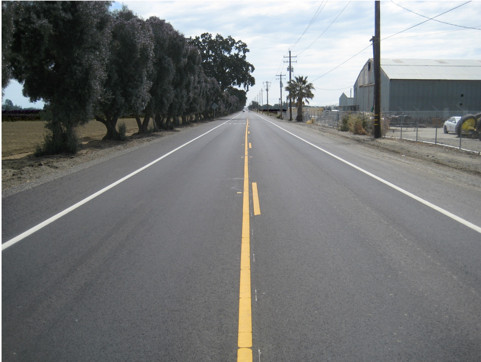
CR 27, Bike Lane & Road Rehabilitation – Photo 4
