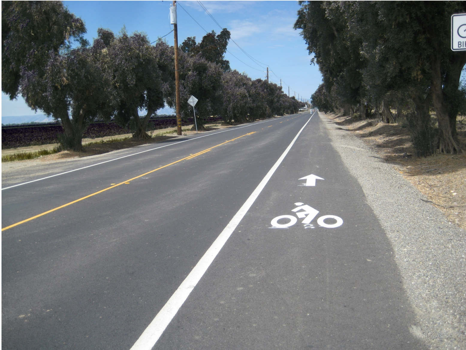
CR 27, Bike Lane & Road Rehabilitation – Photo 3
