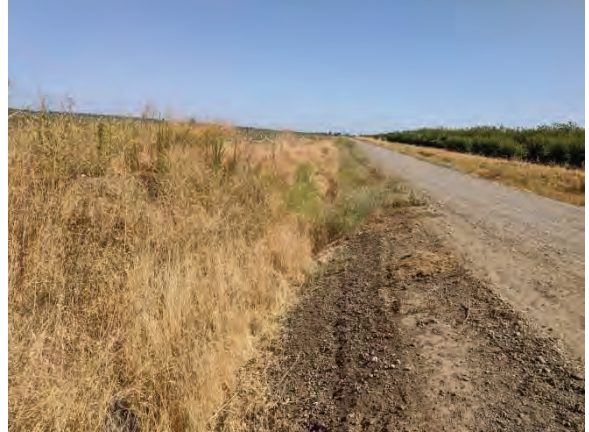
P02 – Upland roadside ditch looking north
