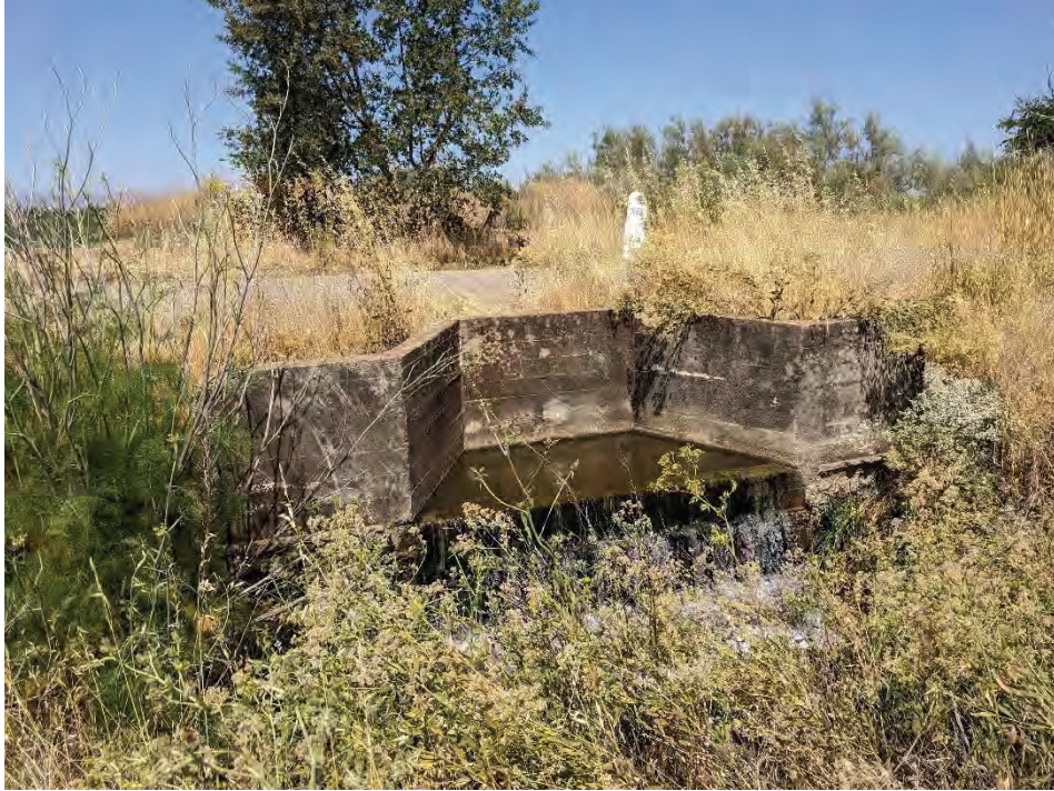
Overview of the Union School Slough diversion channel.
