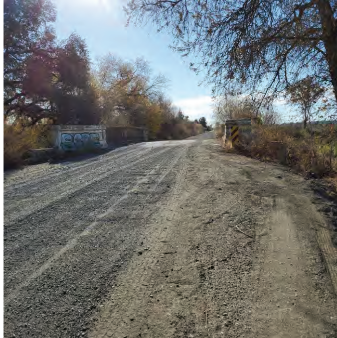
Figure 5. Overview of the bridge approach, viewing south
