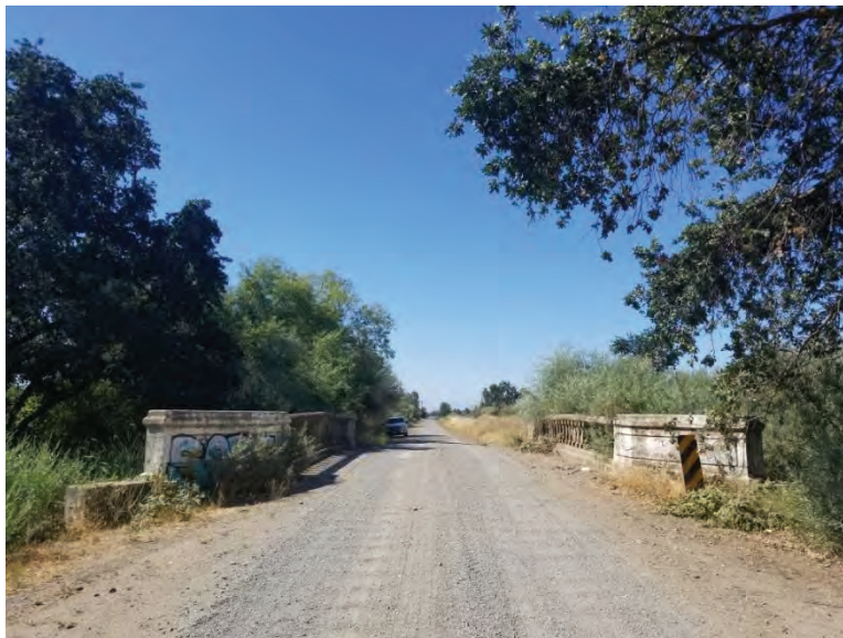
Overview of Union School Slough Bridge. Taken facing south.
