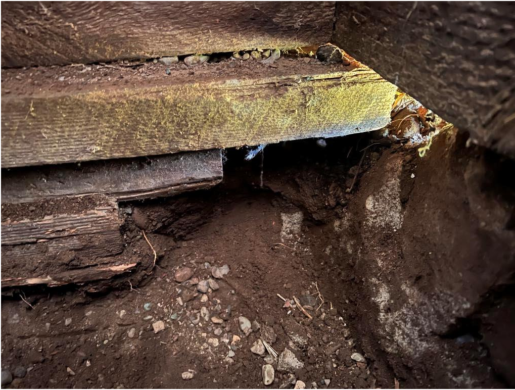
Figure 3: Start of girder
