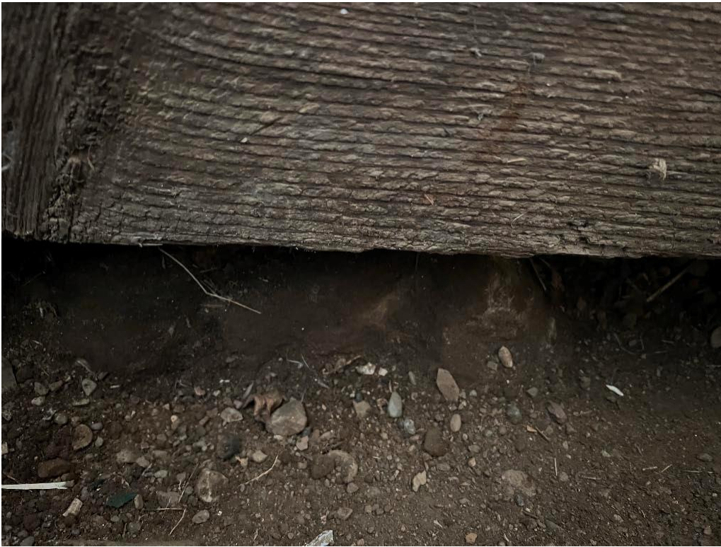
Figure 4: Sandstone support of eastern sill plate
