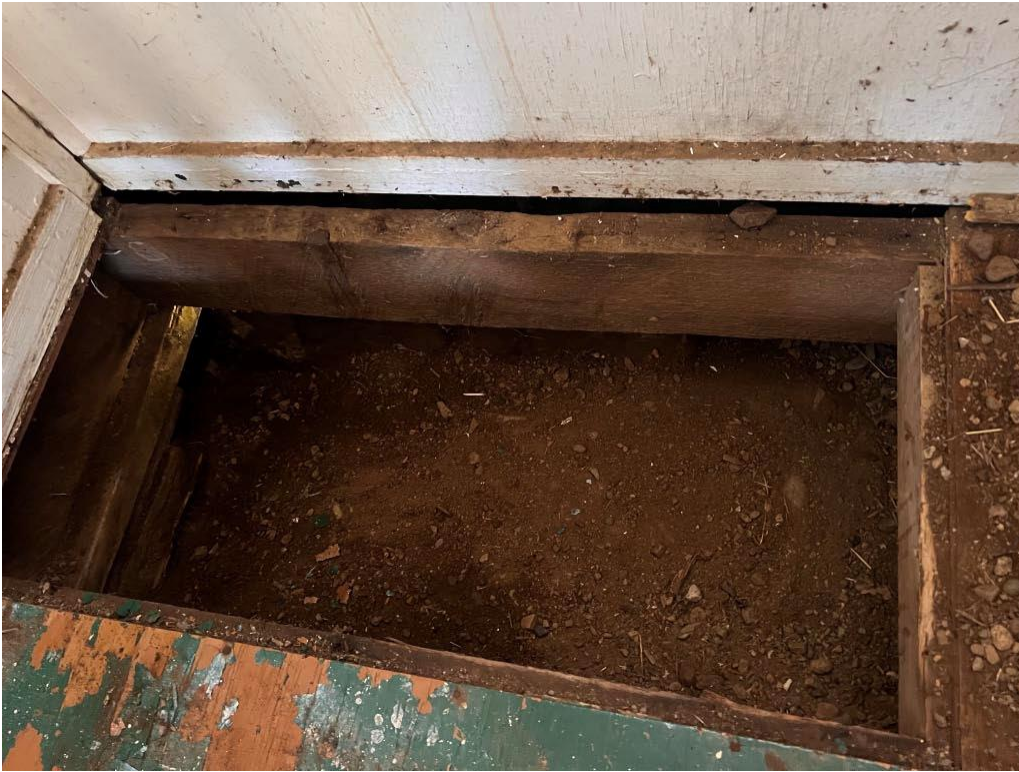
Figure 2: Excavated bay showing eastern most floor joist
