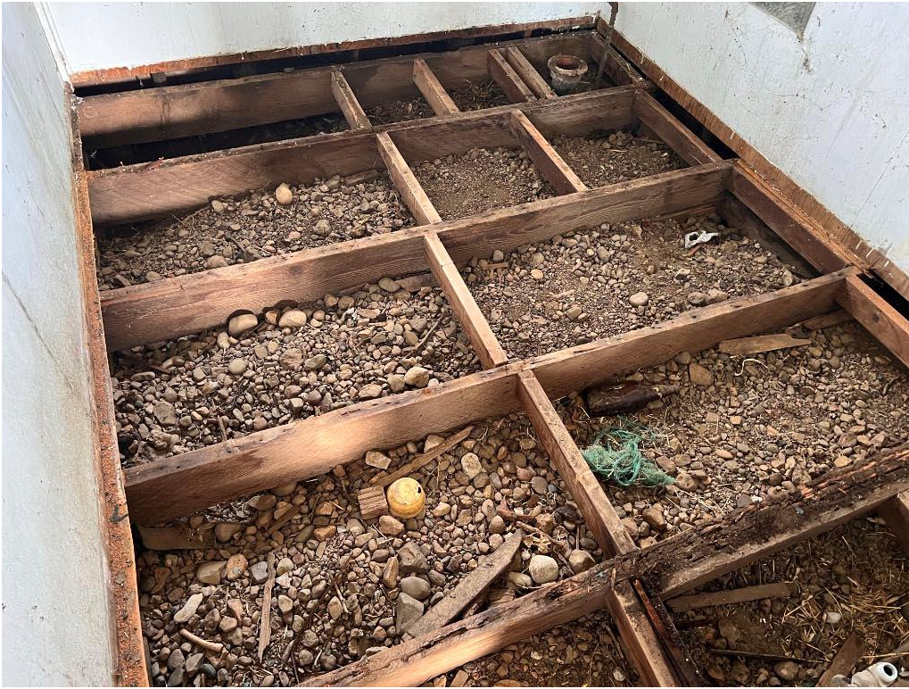
Figure 1: Bathroom floor joists, overview
