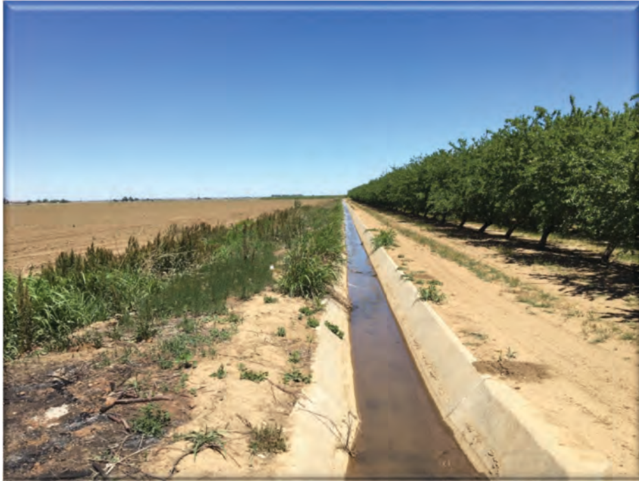
Plate 6. Looking north along the irrigation canal bordering the eastern boundary of the project. This is also a concrete-lined permanent water conveyance feature.
