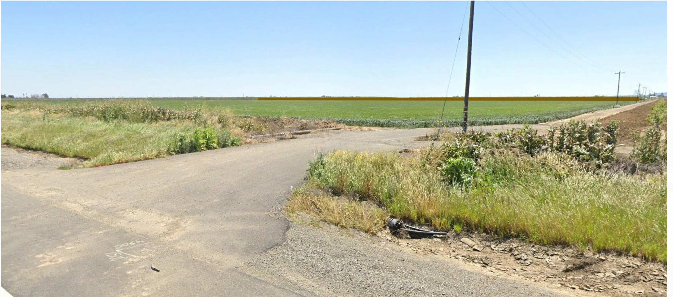
Draft simulated view of revised project configuration. State Route 16 – Looking southeast at the proposed Project site.
