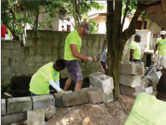
Steve and ISF team building a flood-protection wall.
