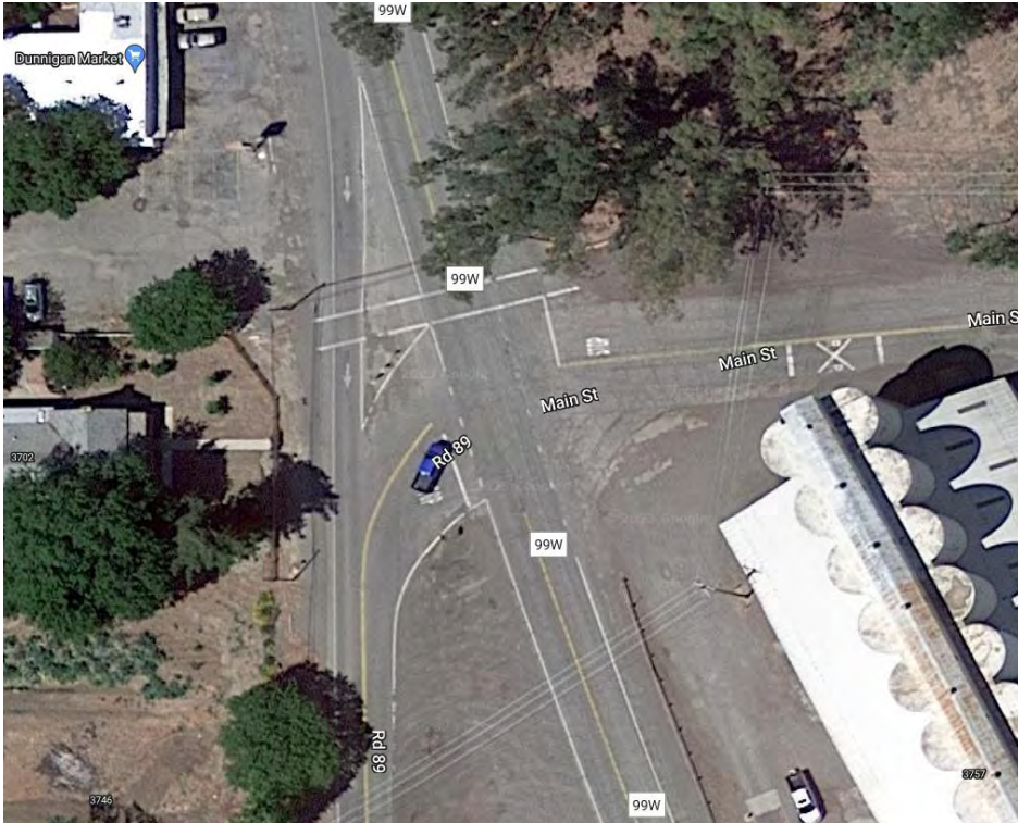
Figure 13. Main Street, CR 99W, CR 89 Intersection
