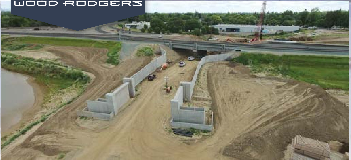
City of Sacramento – McKinley Village Underpass Floodgate Installation
